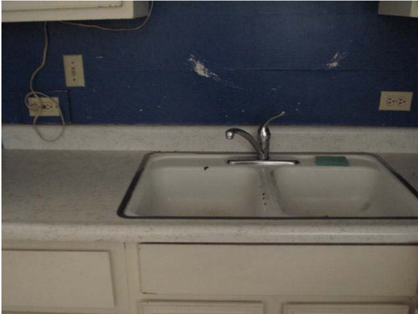
Existing Kitchen Counter and Sink
