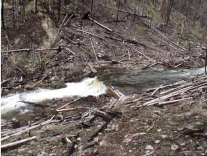
**Figure G-5.** Fish barrier constructed mostly of logs and rocks in 2008 to temporarily isolate East Fork Specimen Creek for restoration of native westslope cutthroat trout. Vegetation is recovering following the Owl Fire, which burned the watershed (including the barrier site) in 2007.
