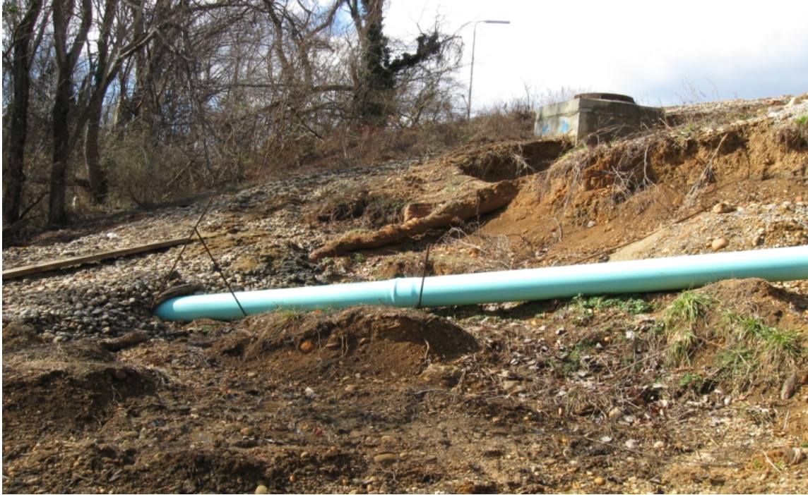
Figure 3 - Exposed drainage piping and unstable slope embankment looking northeast. Soil piles in wooded area at bottom of embankment.
