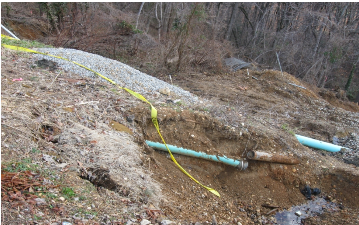
Figure 3 - Exposed drainage piping and unstable slope embankment looking northeast. Soil piles in wooded area at bottom of embankment.
