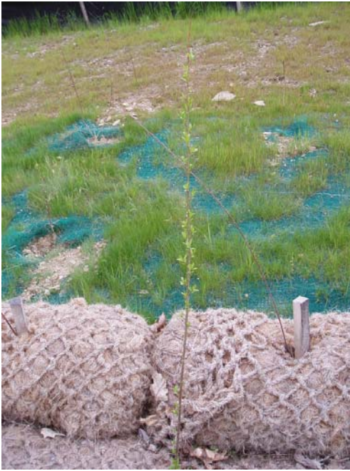
Figure 4 - 1. Coir log used as check dam / runoff dissipater (2010) (MBD Coir Log.JPG)
