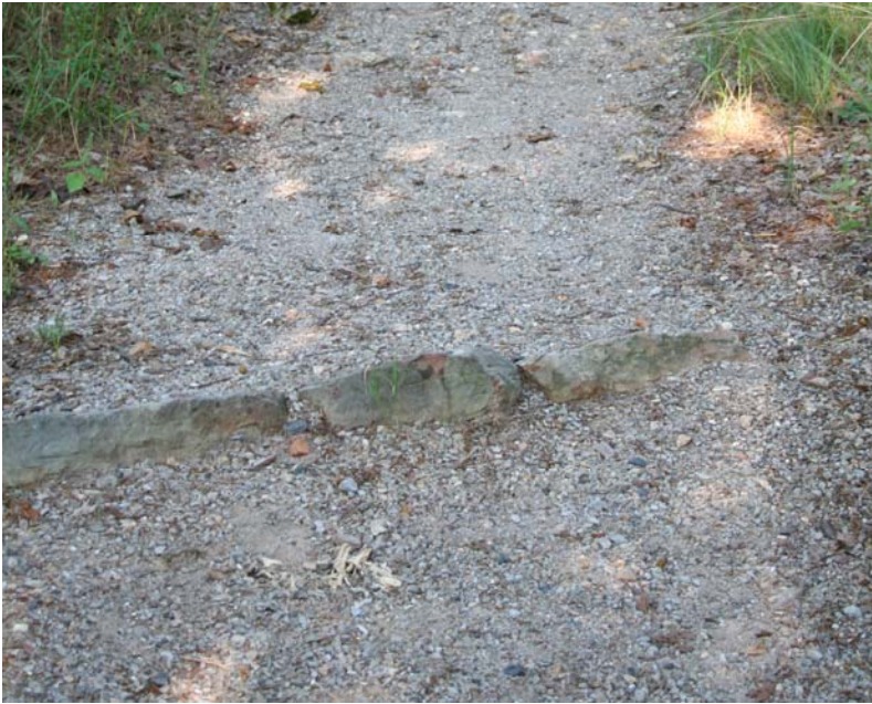
Figure 4 - 3. Stone Water Bar (2010) (MBD Stone Water Bar.JPG)
