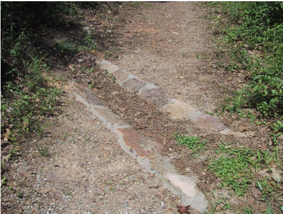
Figure 4 - 2. Stone Drainage Channel (2010) (MBD Stone Drainage Channel.JPG)
