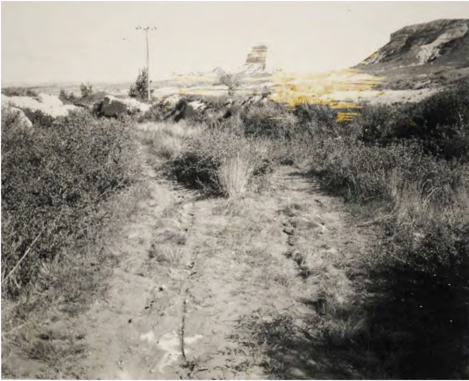
Figure 2 - 34. Sod planted in ruts to stop erosion (c. 1971) (source: SCBL Archives) (DSC_0270.JPG)
