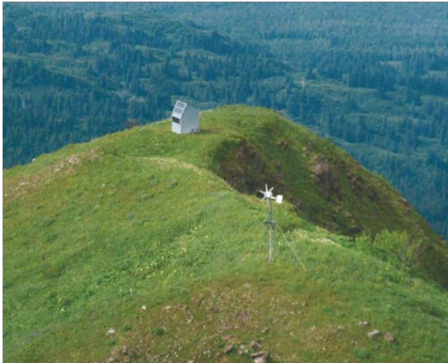
Figure 2-5. Existing Geophysical Institute wind generator and equipment shelter at Deception hills site
