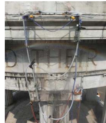
Water mist cleaning
