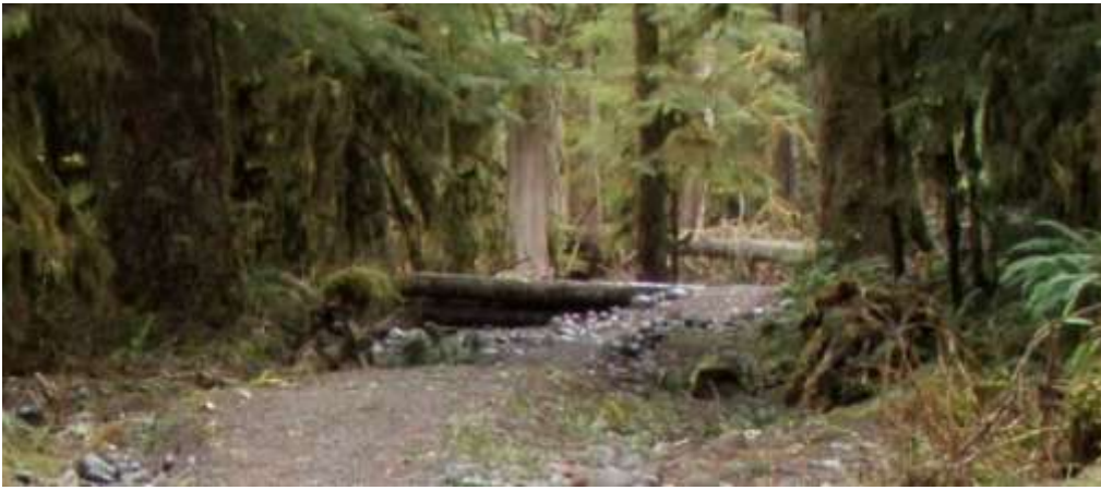
Figure 10: Gravel covered log hump
