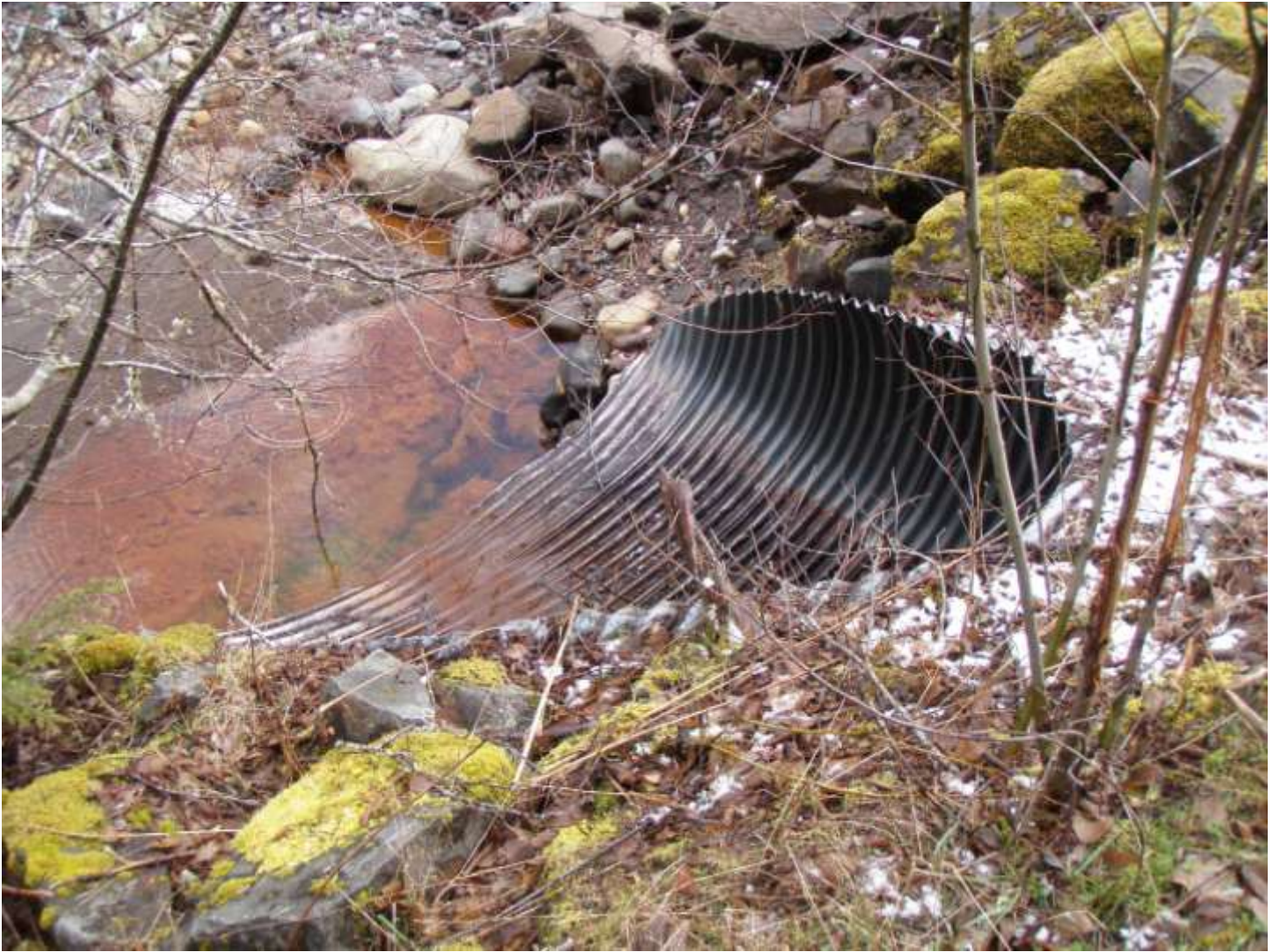
Figure 20: Hanging culvert near “Magirl channel”
