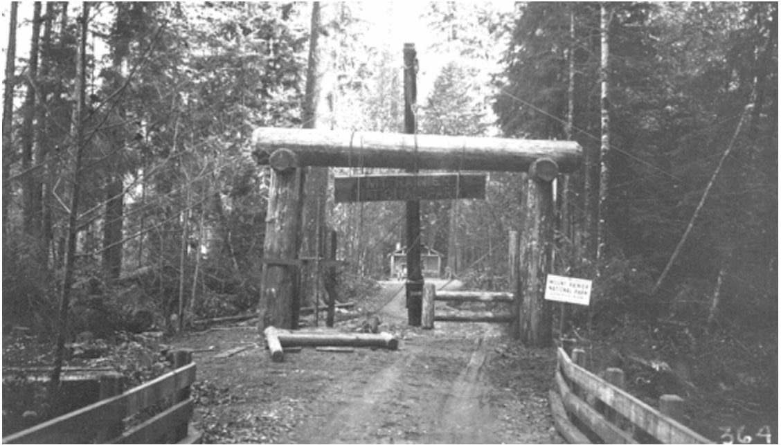
History #10: Historic photograph, looking east, showing the Carbon River Arch under construction, c. 1933 (Photo Number: ps3649, MORA Archives).
