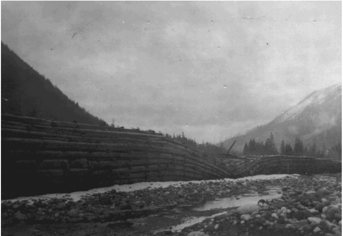
History #6: Log cribbing constructed along the Carbon River, c. 1925 (Photo Number: twc586, MORA Archives).
