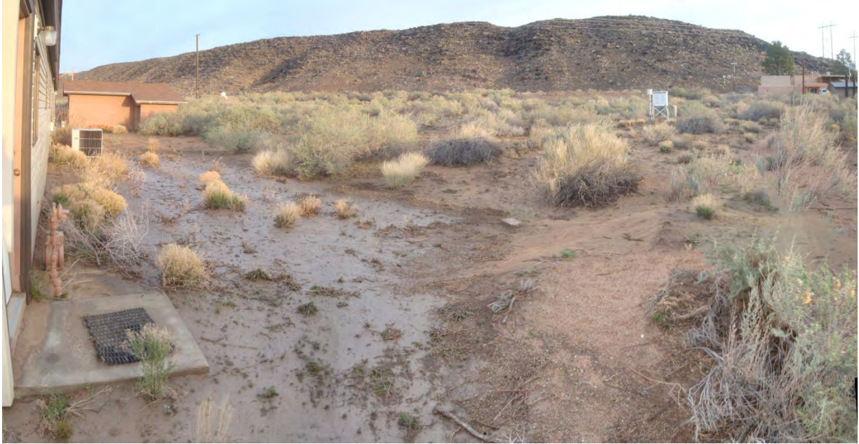
Figure 6. Stormwater Drainage Pooling Behind the Lava Shadows Annex
