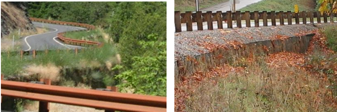
Figure 2.2 – Examples of Retaining Walls. Left wall is 10 to 15 feet in height, well vegetated. Right wall is 3 to 6 feet in height with less vegetation
