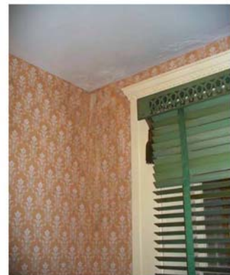
Figure 2. Recently Installed Wall Paper and the Ceiling Plaster and Paint are Damaged as the Result of the Leaking Downspout Outside
