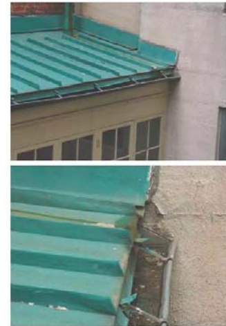
Figure 3. Gutter is Sagging, Full of Debris and does not Slope Toward the Downspout
