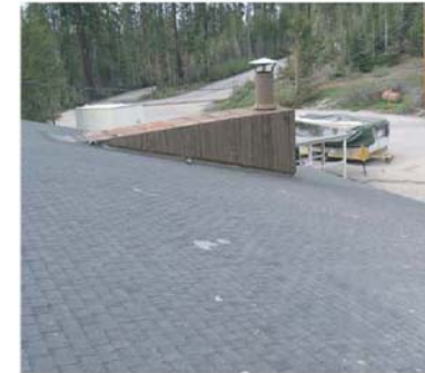
B3010-01: Roof B1 looking northwest.
