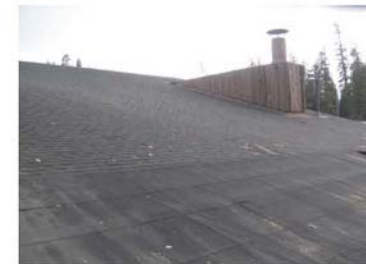
B3010-05: Northern portion of Roof B1 with cap sheeting.
