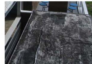
B3010-15: Roof B5 looking south from above.
