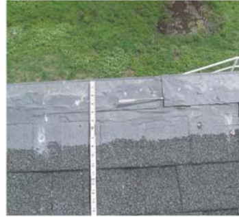
B3010-08: South eave with flashing.
