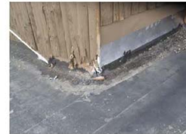
B3010-04: Metal flashing at south wall of Winter Club Addition.
