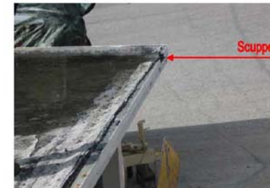
B3010-14: Edge flashing and scupper of Deck B2.
