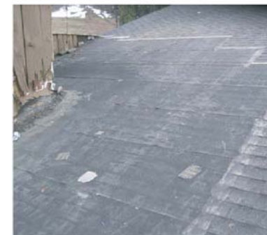
B3010-03: Patch area of Roof B1.
