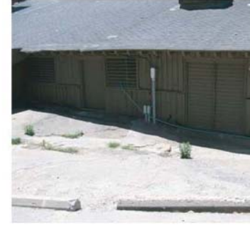
B3010-09: Rafter tails at the north edge.
