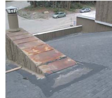
B3010-02: Roof B1 looking northeast.
