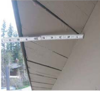
B3010-07: Eave of Roof B1.
