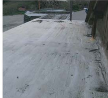
B3010-11: Roof B2 looking north.
