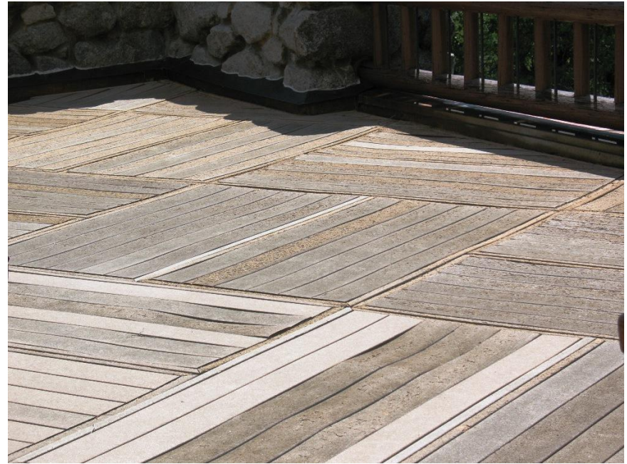
Photo #6 - Uneven finish, sagging, and cracking TREX boards.
