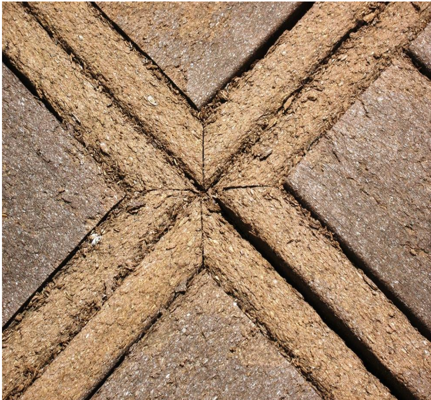
Deterioration #1 – Note the eroded particles of the TREX material. These particles are causing drainage blockages under the decking system.
