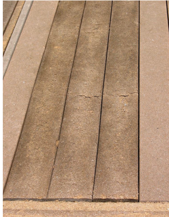
Deterioration #2 - Cracking and uneven surfaces.
