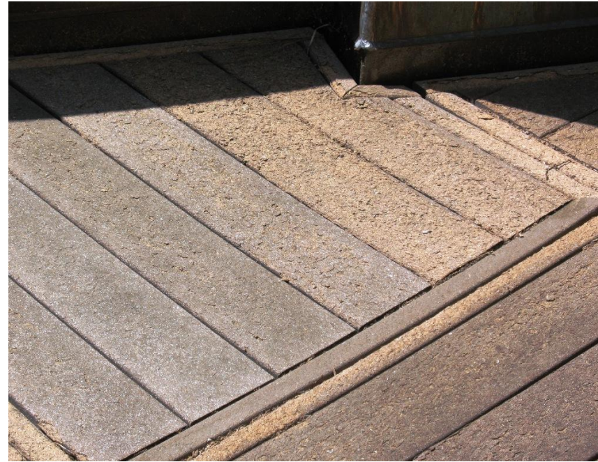
Deterioration #4 – Uneven surface, eroded material, uneven finish.
