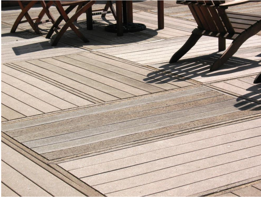
Photo #5 - Note the panel design and uneven finish.
