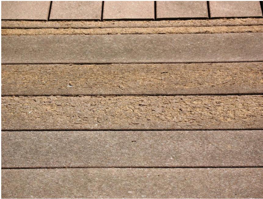
Deterioration #3 – Eroded flaking material.
