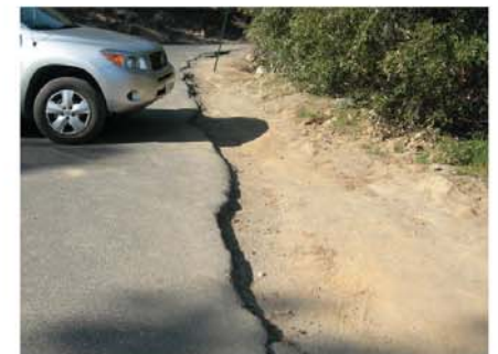
Soil erosion and broken asphalt edge
