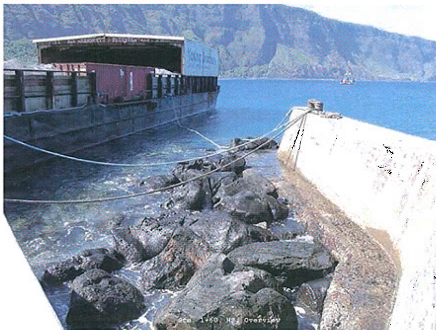
Barge and moor lines to breakwater. Note displaced armor stones resting in berthing basin adjacent to breakwater.
