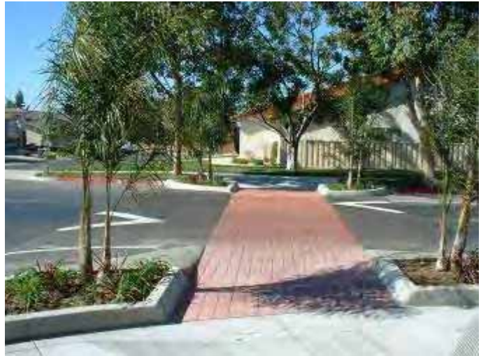
Sample photo of a raised crosswalk made of brick. The materials and markings used on Moors Road may vary.
