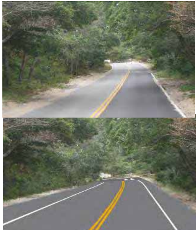
Top: Existing view, looking southeast along Moors Road at access point 2. Bottom: Simulation of widened shoulders and a raised crosswalk in the same location.
