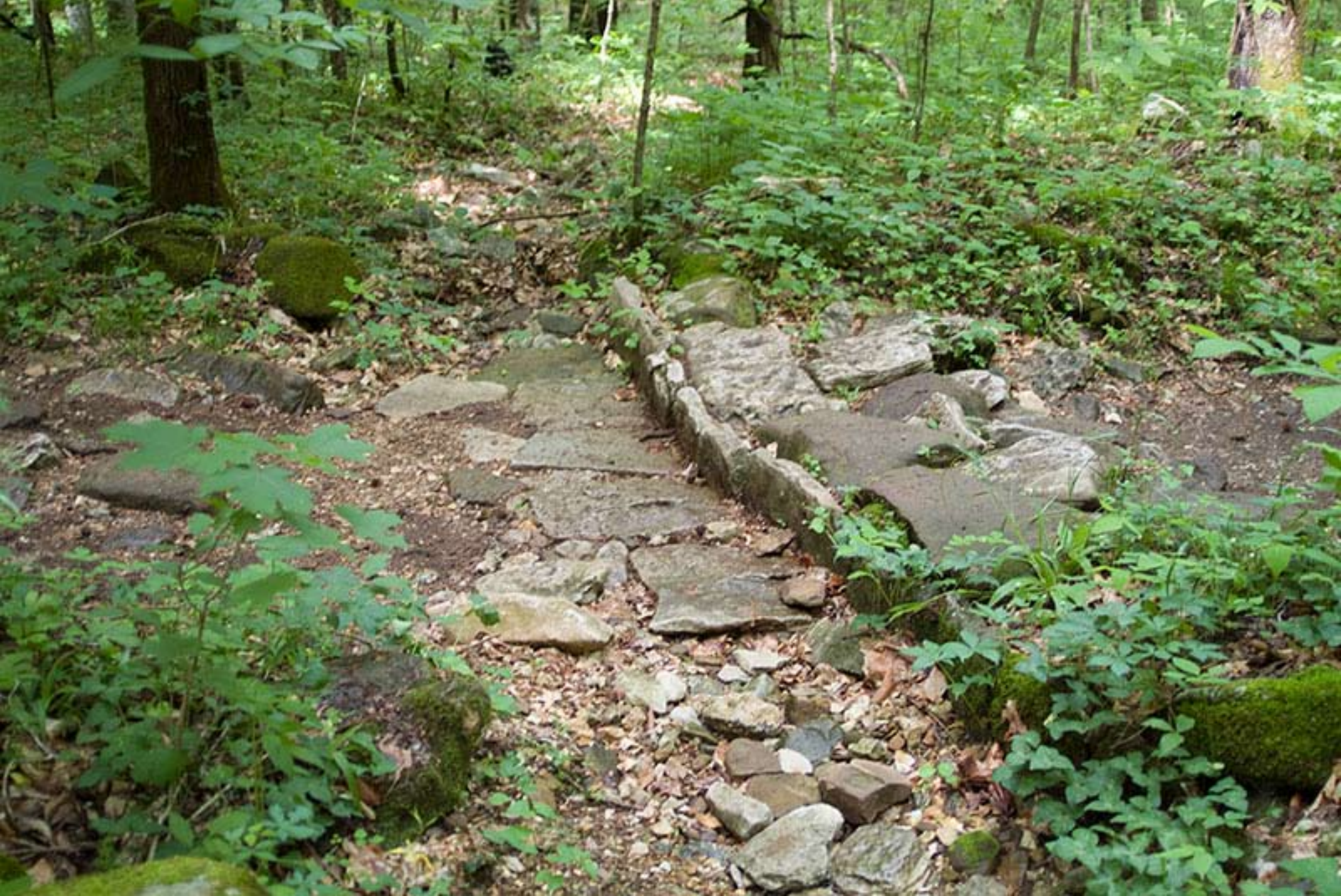
Flagstone drainage crossing on Lost Valley Trail.
