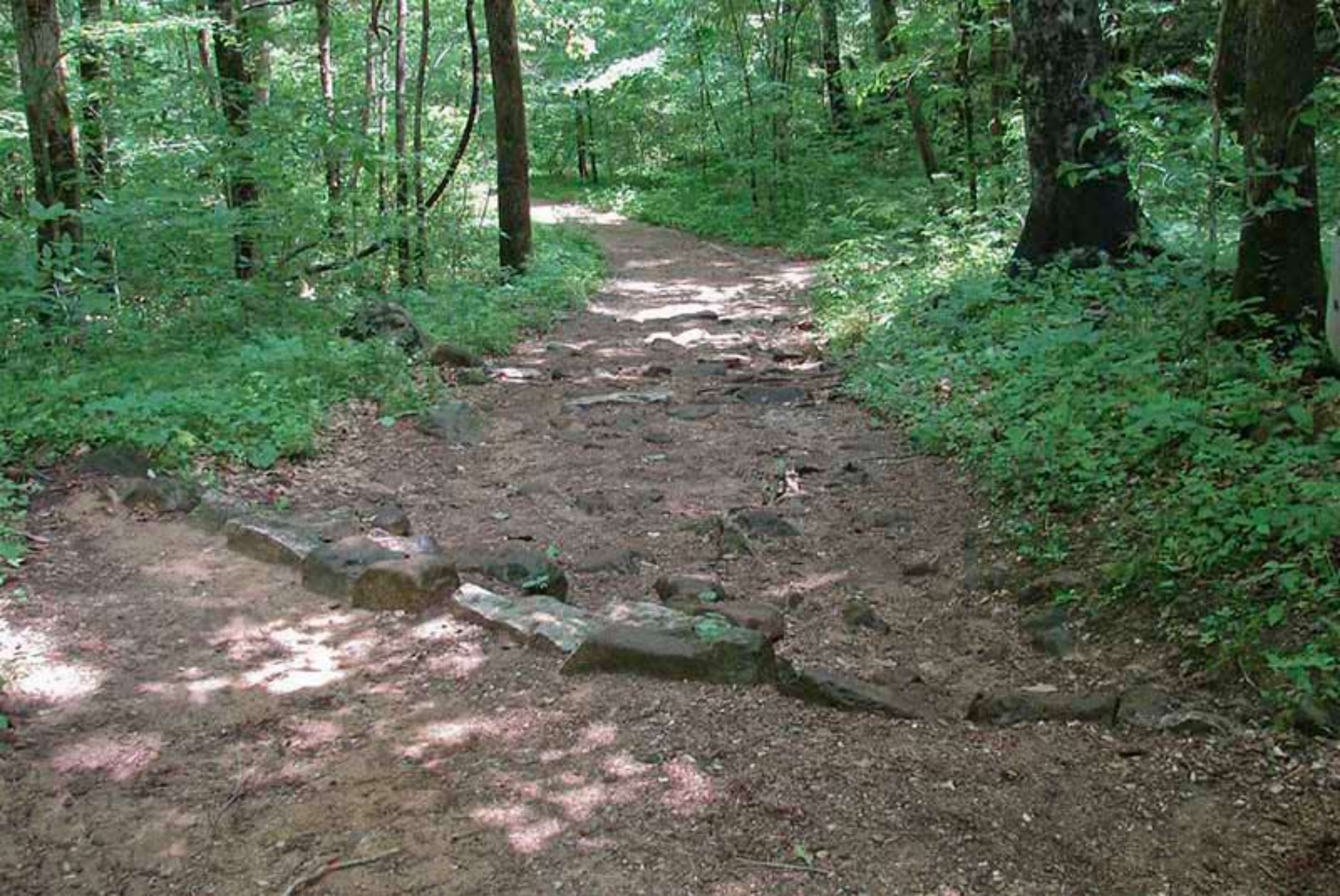
Drainage crossing/safety (trip) hazard on Lost Valley Trail.
