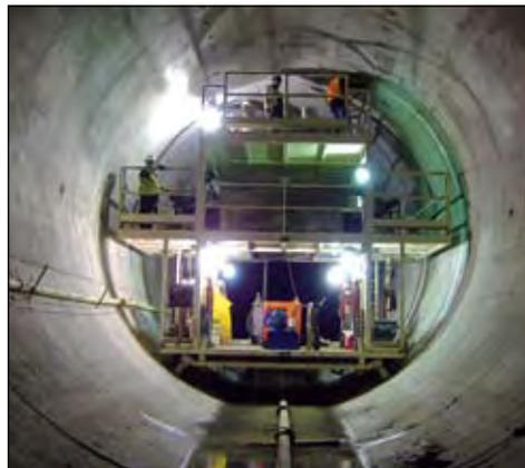
CSO control involves the construction of miles of subway-size tunnels 150 to 250 feet underground, like this one in Atlanta.
