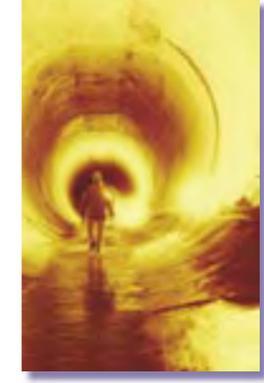
CSO underground tunnels will be equivalent to a 10-mile long sub-way tunnel, 25 feet in diameter.
