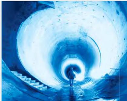
The combined sewer overflow (CSO) control program includes the construction of miles of metro-size tunnels 150 to 250 feet underground.
