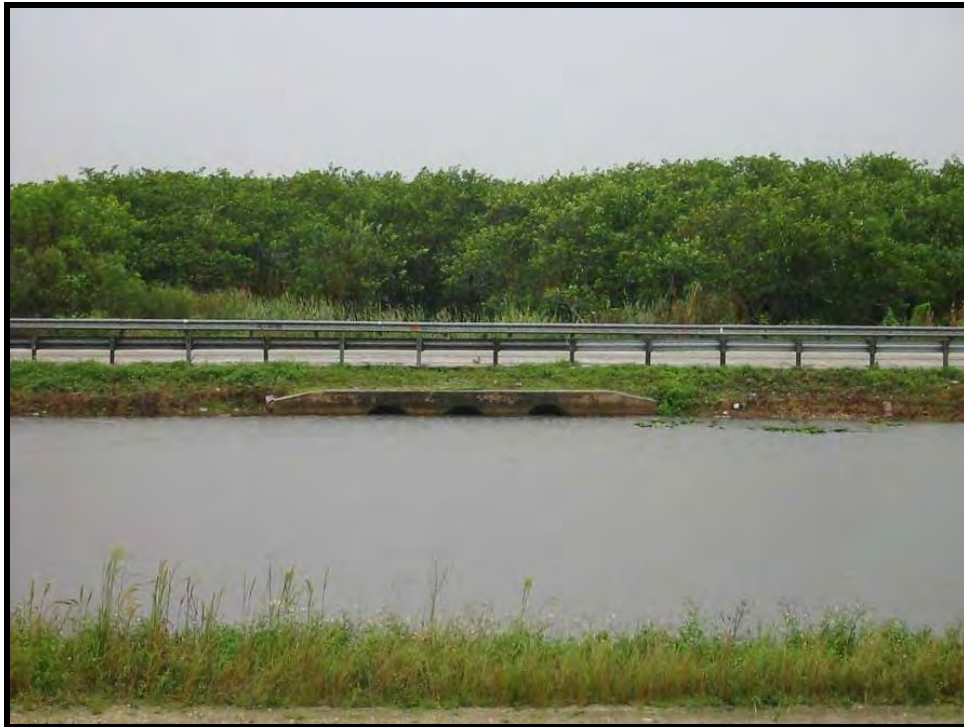
Figure 2 – One of 19 Sets of Existing Culverts, Looking South from L-29 Levee
