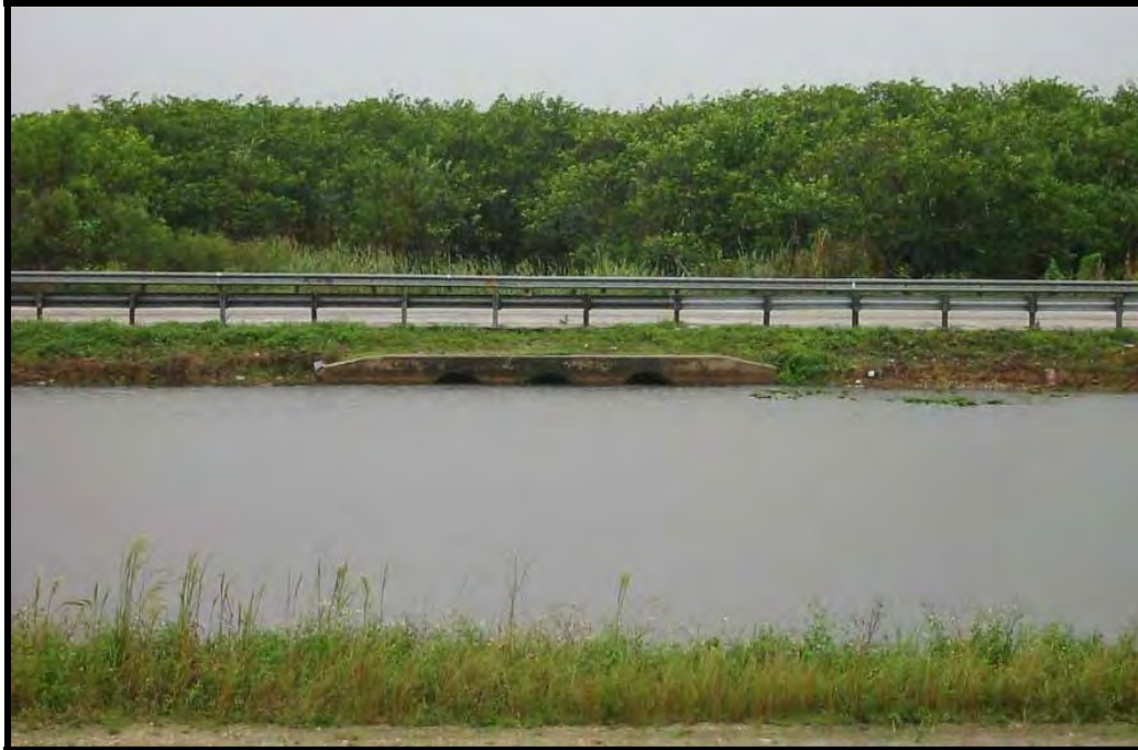
Figure 3-21 – One of 19 Sets of Existing Culverts (Facing South from L-29 Levee)
