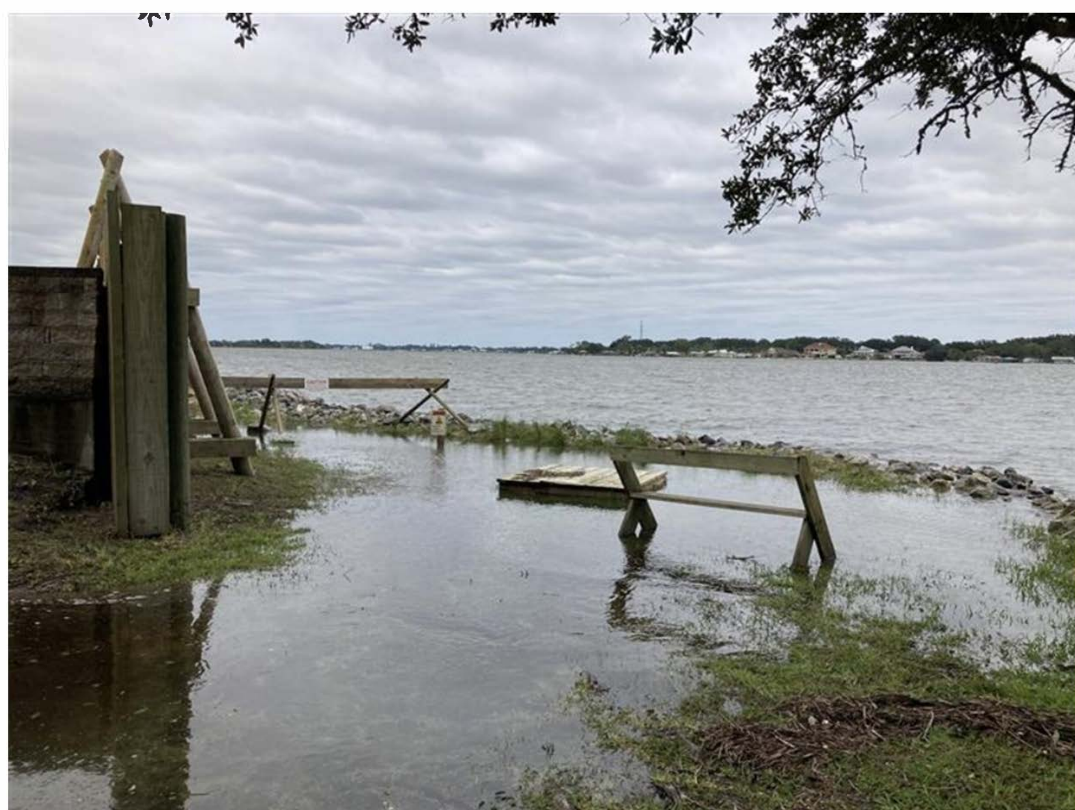
Figure 3. Figure 3 Flooded Walkway on NE corner of Exhibit
