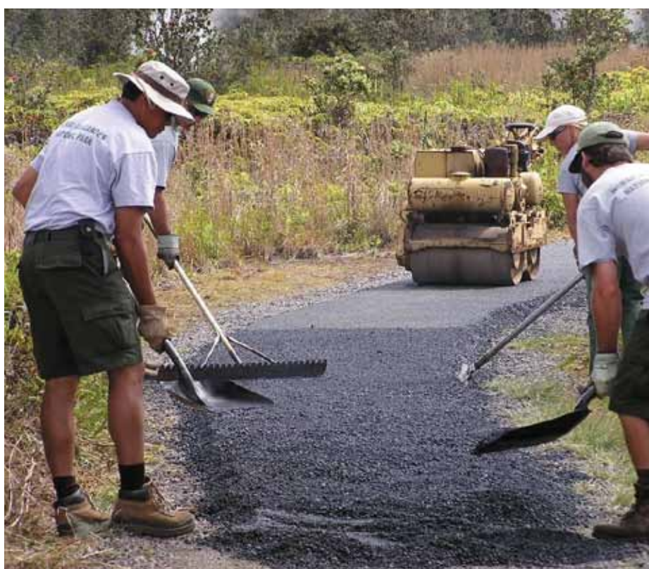
Maintenance crews paving accessible trail to Sulphur Banks
