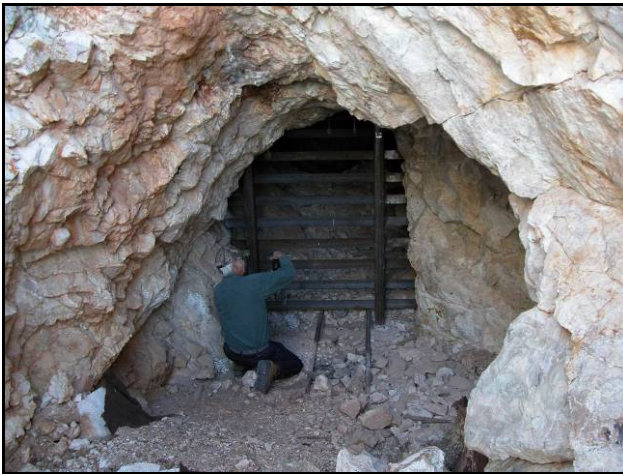
Photo 19. Adit closed with a bate gate.
