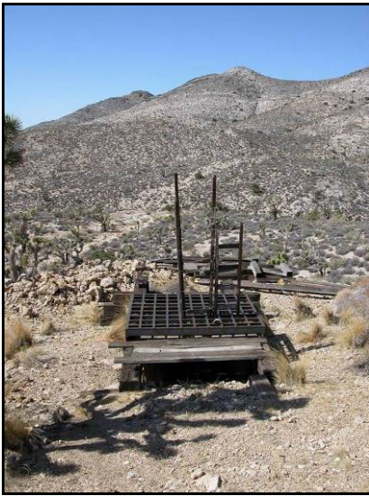
Photo 9. Bat gate over vertical shaft.
