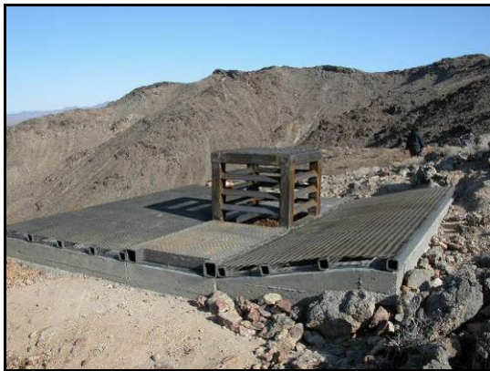
Photo 15. Shaft closed with combination grate, bat cupola and concrete footing. The footing acts as a deterrent for desert tortoises.
