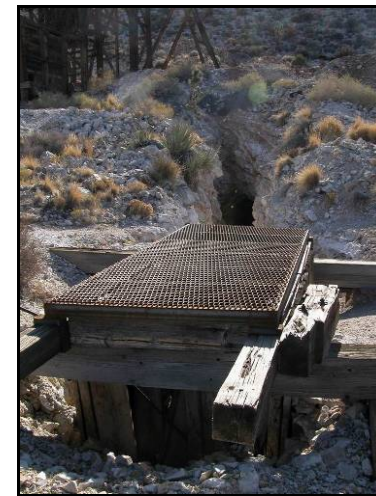
Photo 24. Grate over a vertical shaft.
