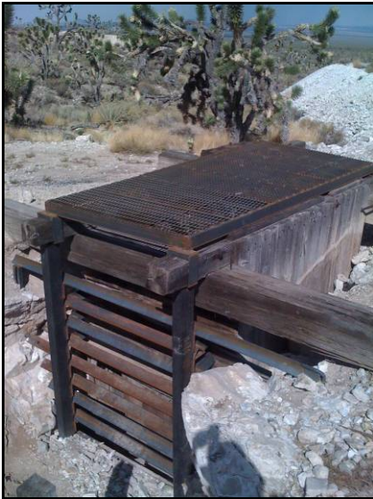
Photo 25. Combination bat gate and grate over a vertical shaft.
