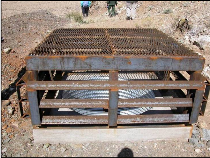
Photo 1. Bat cupola over a vertical shaft.
