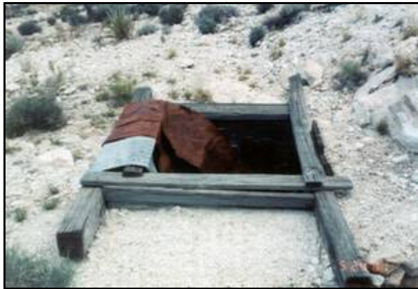
Photo 23. Unclosed vertical shaft.
