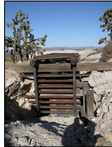
Photo 22. Closed vertical shaft with bat gate.
