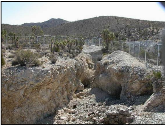
Photo 7. Trench mine with shafts and adits, with permanent fencing.
