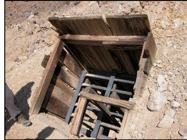
Photo 14. Recessed bat gate in a decline. Note minimal disturbance in area surrounding the opening, and preservation of features.
