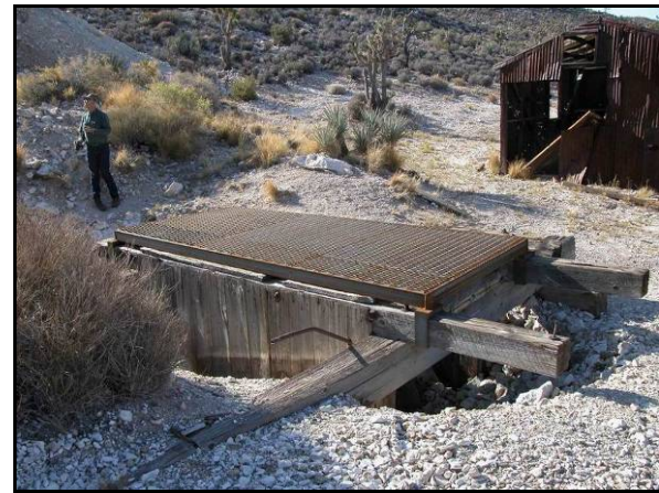
Photo 10. Grate over vertical shaft
