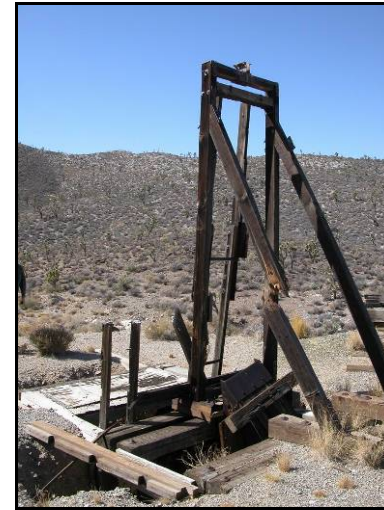
Photo 26. Unclosed vertical shaft with head frame.
