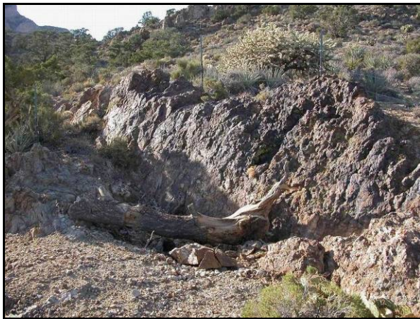
Photo 11. Completed polyurethane foam plug.
