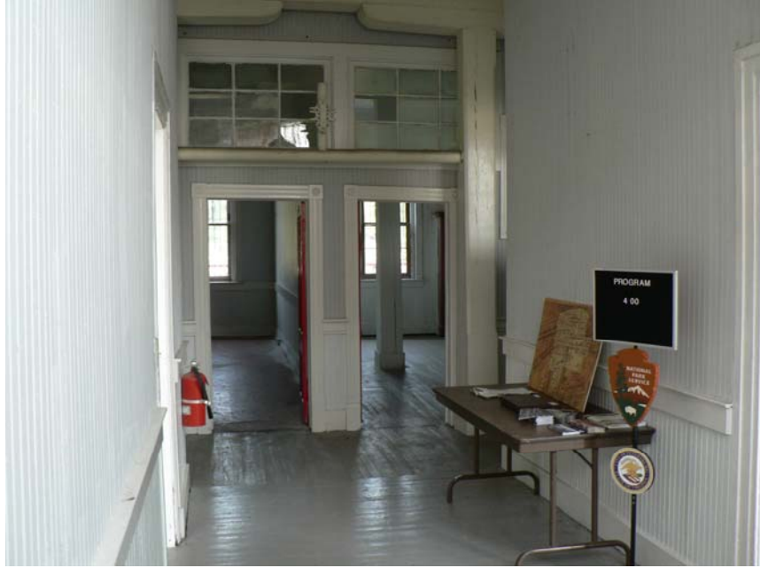
5. Interior Hall, South Side Depot, Petersburg, VA
