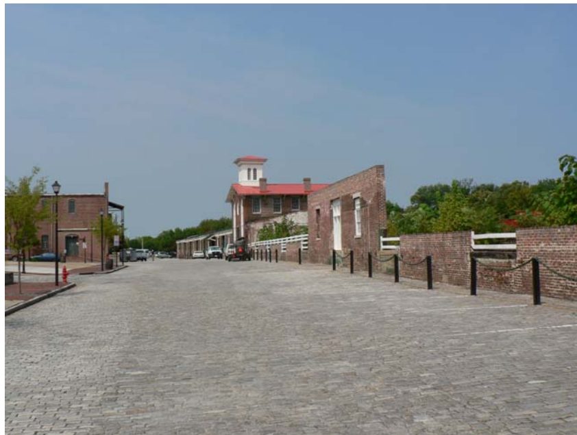
4. East Wing (Damaged in 1993 Tornado), South Side Depot, Petersburg, VA
