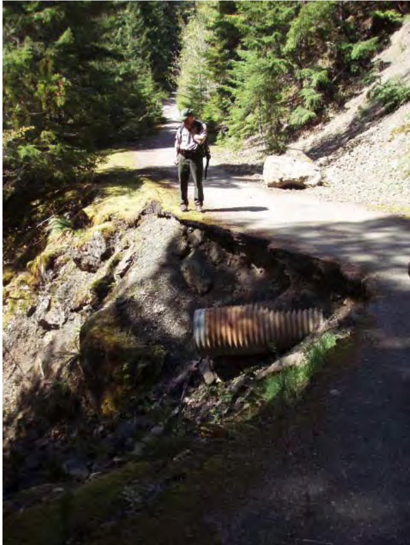
**Photo 9: Culvert along the Boulder Creek trail.**
