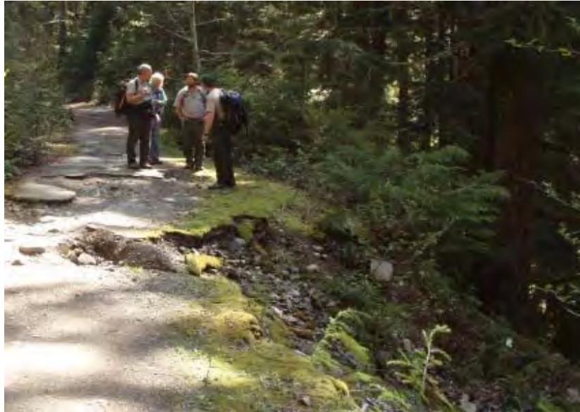
**Photo 10: Deteriorating asphalt along the Boulder Creek trail.**
