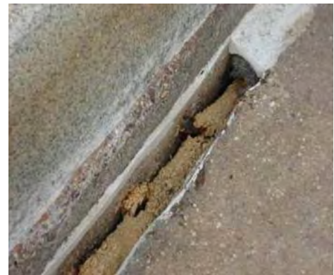
Figure 2.4 – Deterioration of the joints at the Reflecting Pool granite coping
