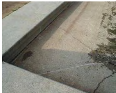
Figure 2.4 – Deterioration of the joints at the Reflecting Pool granite coping
