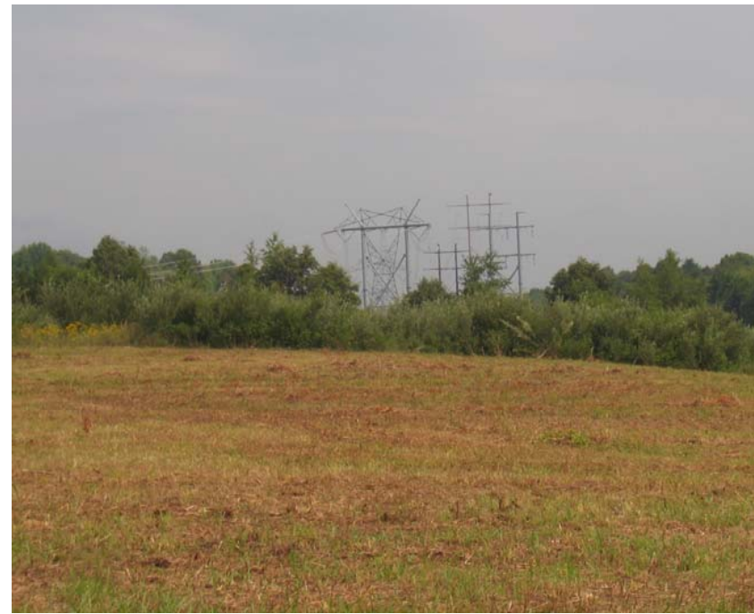
Both types of high voltage power lines now existing on the battlefield are shown above. Both types average approximately 100 feet in height.
