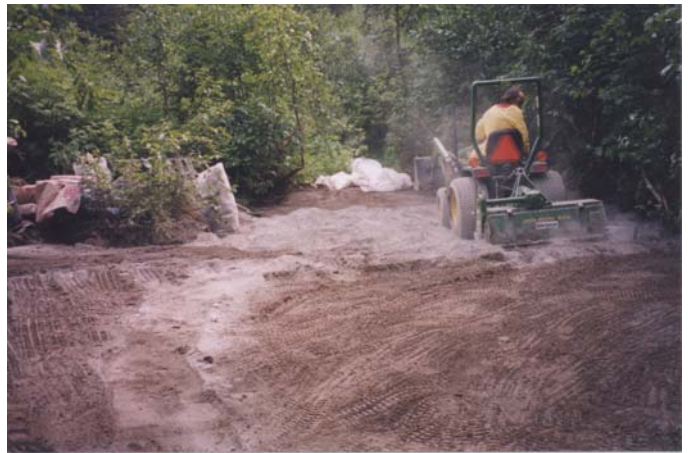
Photo 4. Rototiller mixing cement with tailings.
