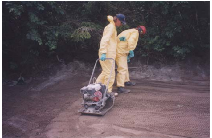
Photo 5. Compacting tailings/cement mixture.
