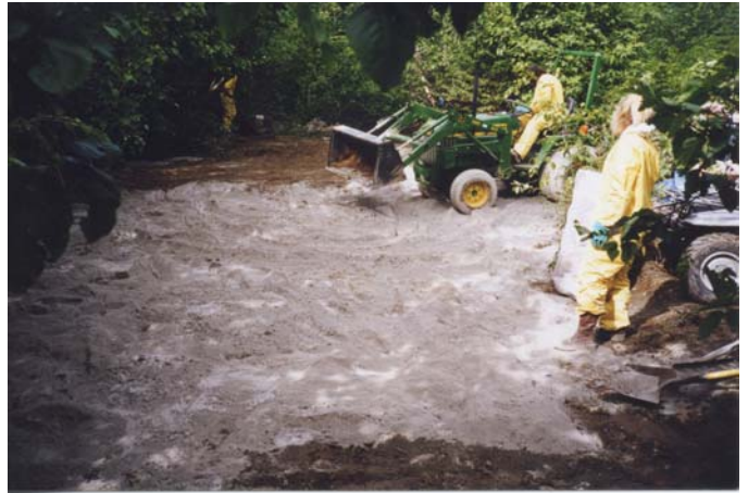
Photo 3. Application of Portland cement to surface of Pond D- July 1998.
