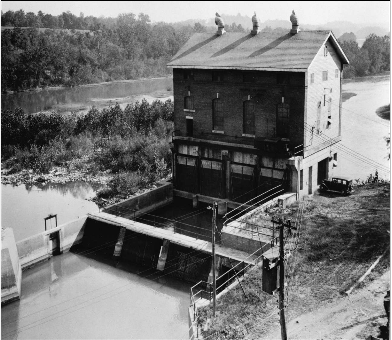
PHOTO NO. 9: HISTORICAL VIEW OF DAM 5 HYDROELECTRIC PLANT, CIRCA 1933. View shows powerhouse, forebay and river. Source: Historic American Buildings Survey; photograph provided by Potomac Edison Company.
