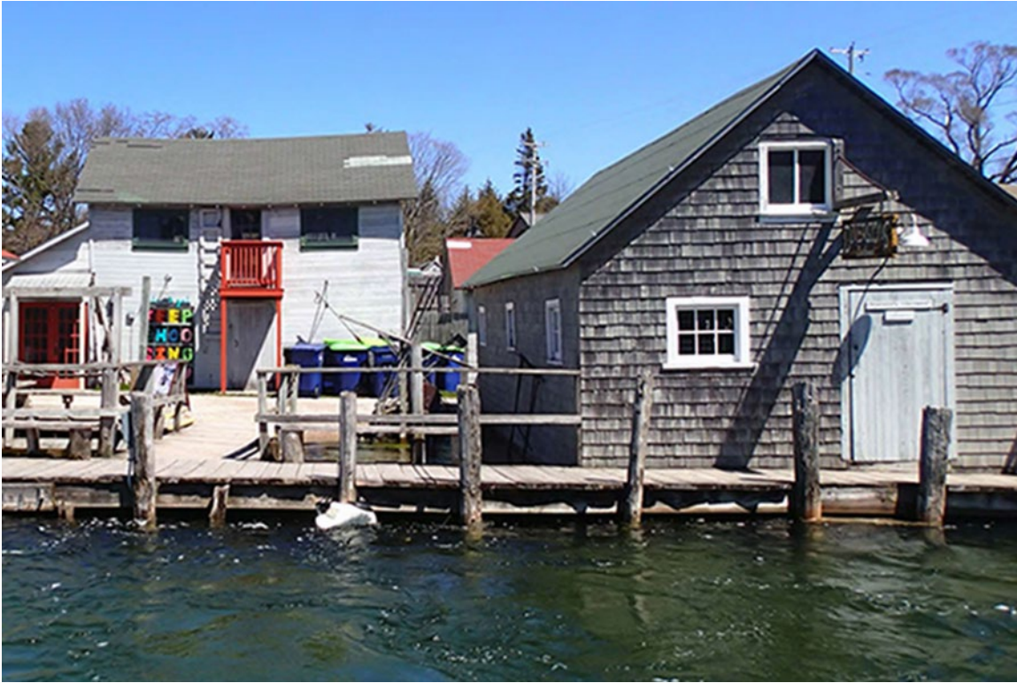
Figure 44. Early photos of “Building 7” (right) in Fishtown Historic District, Michigan (NR Ref. No. 10000676), show a wood shingle roof, later replaced with hexagonal multicolored asphalt shingle in the summer of 1934, and then by green asphalt rolled material during the 1950s. Nevertheless, Building 7 retains integrity of location, setting, design, feeling, and association. (Amanda Holmes)
