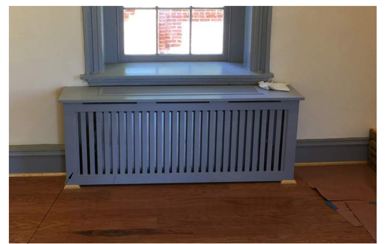
THIS EXAMPLE DEMONSTRATES A CUSTOM ENCLOSURE FOR A FAN COIL UNIT. THE DESIGN INTENT IS TO BE COMPATIBLE WITH EXISTING HISTORIC ROOM FINISHES. SIZE AND LOCATION TO BE COORDINATED WITH FURNISHING AND EXHIBIT LAYOUT IN NEXT DESIGN PHASE.
