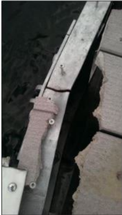
Failed connection at main truss.
