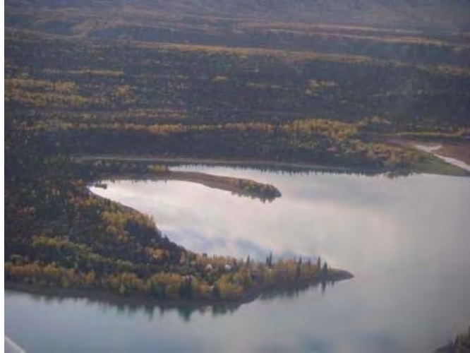
Photo 1: Hardenburg Bay, looking south from Lake Clark, showing some existing structures (NPS)
