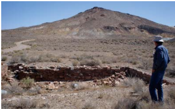
Foundation remains, NPS photo
