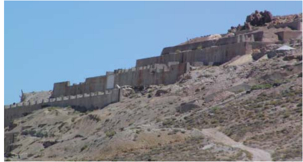
Foundation of 100 Stamp Mill
