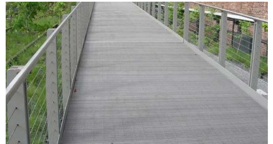
This metal decking has been used in at High Line Park to provide a “see-through” look while remaining ADA compliant.
