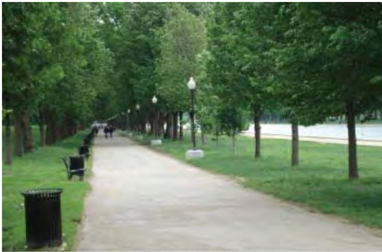
SIDEWALKS UNDER THE ELMS ARE IN DISREPAIR, AND MUST BE REPLACED
