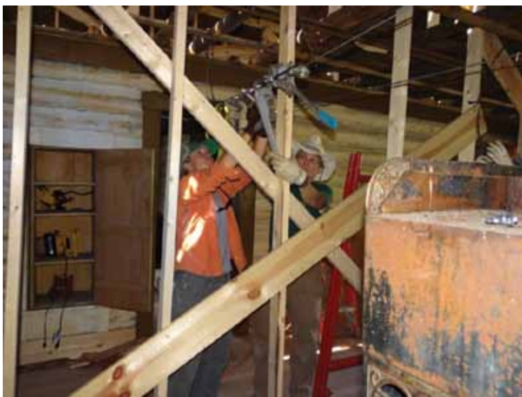
Figure 12.6 —Installing emergency roof supports in the main lodge, OTO Dude Ranch, Custer-Gallatin National Forest. Routine and emergency projects to stabilize, protect, and maintain historic buildings are likely to increase in a warmer climate (photo by Marcia Pablo, Custer-Gallatin National Forest).
