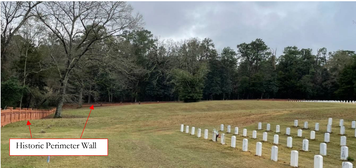
4c: Photo looking south from Section J along the eastern edge of Sections J and Q. This provides a sideview of the sloping drain of Section Q. The historic perimeter brick wall is seen along the east and south sides of Section Q.
