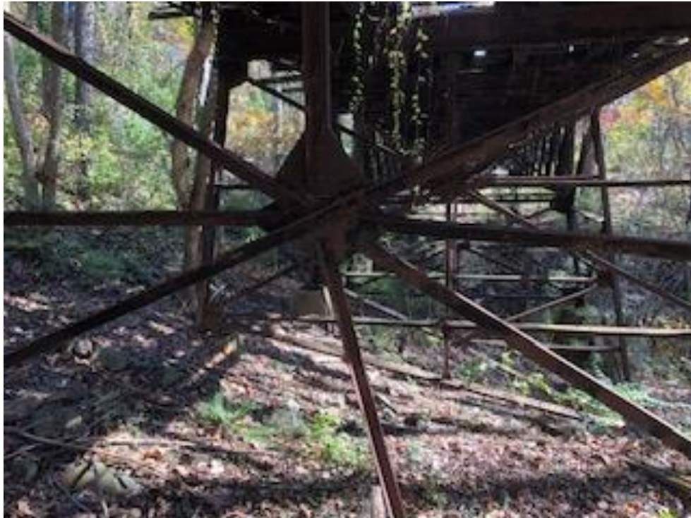
Figure 7: Interior trestle tower bracing with diagonal, horizontal, and vertical beams and chords and polygonal shaped gusset plate
