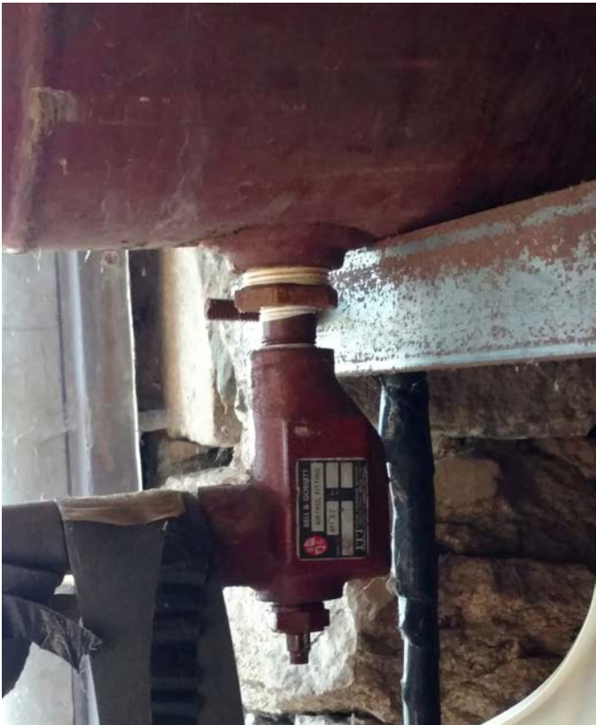
Figure 3.27 Chilled Water Airtrol Tank Fitting M3
