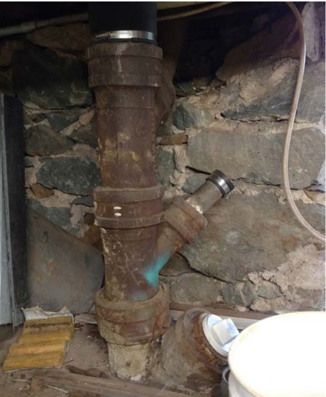
Figure 3.61 Large Amounts of Rust on Sanitary Piping in Unfinished Basement P3
