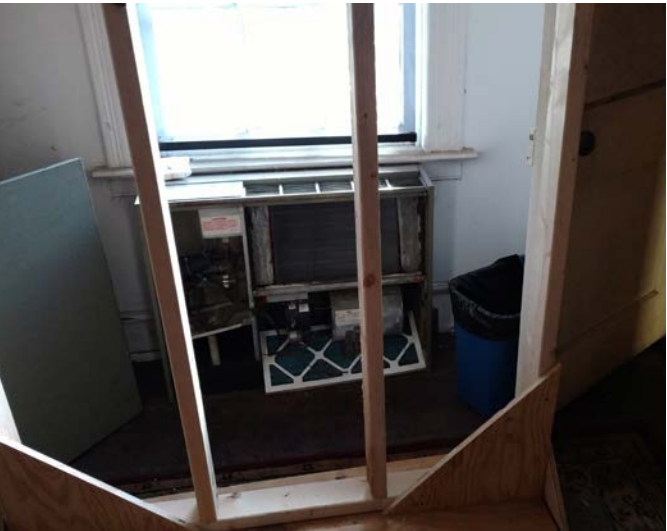
Figure 3.64 Four-pipe Fan Coil Unit serving Office 106 M18
