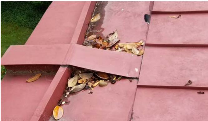
Pooling Water at Roof Expansion Joint
