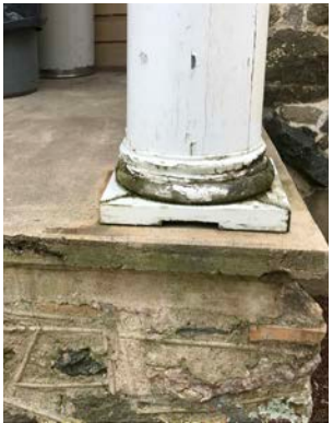
Weathering at Column Base
