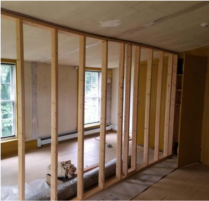
Figure 3.16 Structural Shoring in Dr. Hubbell's Bedchamber [206]
