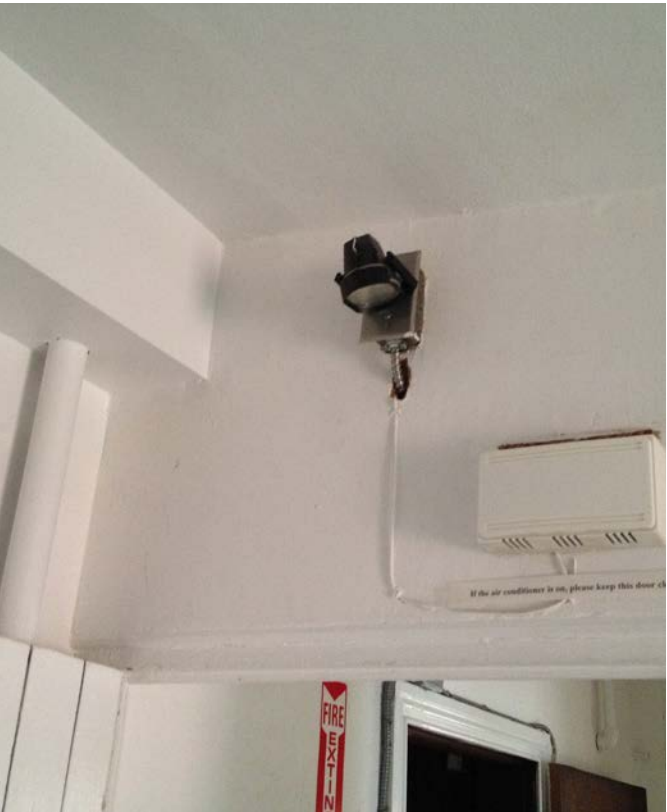
Figure 3.115 Emergency lighting and exit signage deficiencies E8
