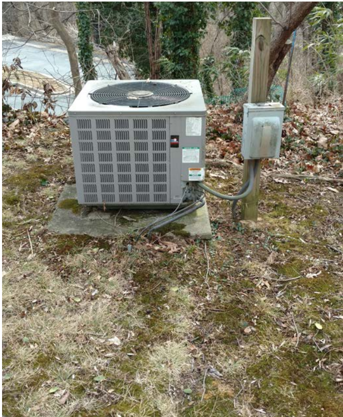
Figure 3.23 Chiller Air-Cooled Condenser M7
