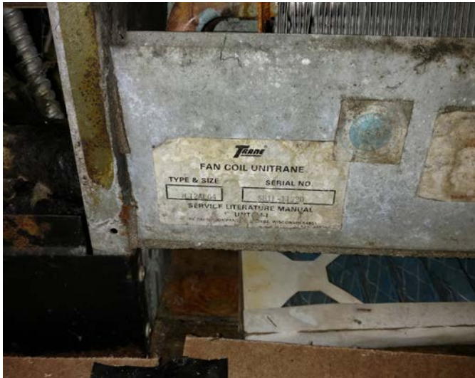
Figure 3.67 Fan Coil Unit Nameplate Data (Visitor Orientation 113) M19
