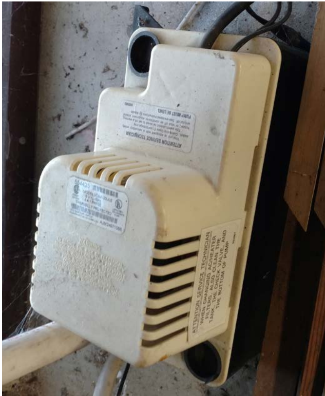
Figure 3.36 Condensate Pump in Unfinished Basement M4
