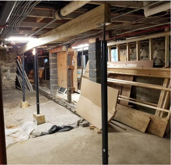
Figure 3.13 Structural Shoring in Unfinished Basement [001]
