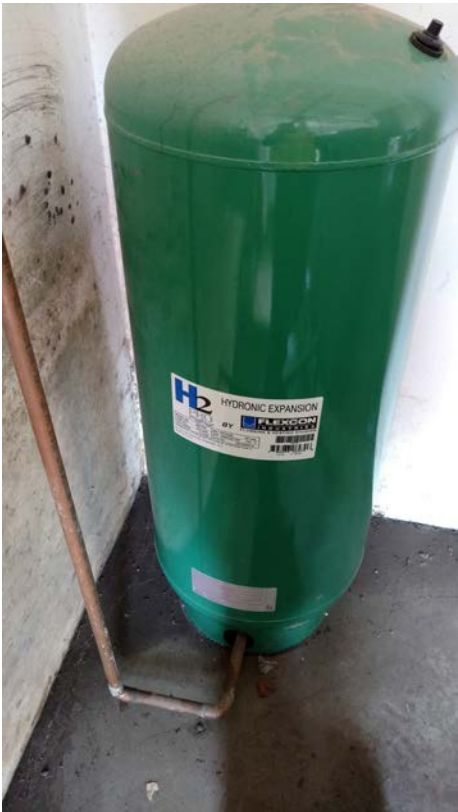
Figure 3.46 Heating Hot Water Vertical Expansion Tank in Boiler Shed M14
