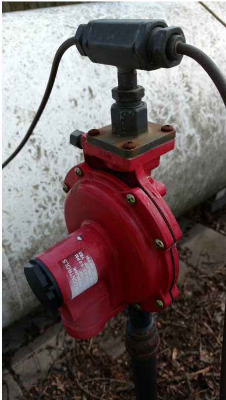
Figure 3.55 Gas Regulator (Outside)
