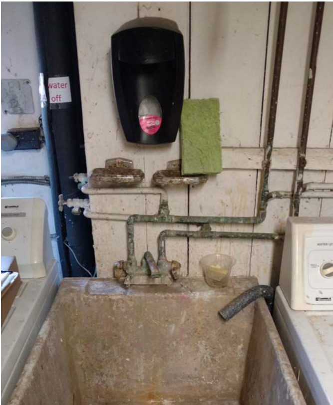
Figure 3.59 Oxidation and Calcium Build-up on Domestic Cold and Hot Water Piping P2
