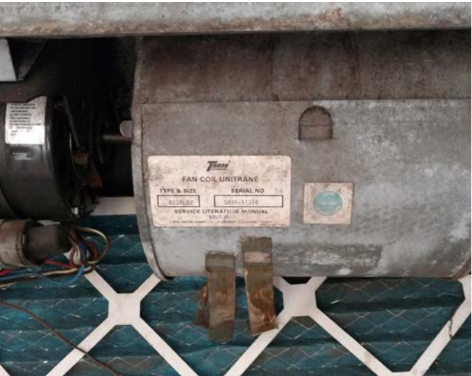
Figure 3.65 Fan Coil Unit Motor and Nameplate Data (Office 106) M18
