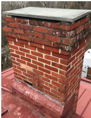
Weathered Masonry and Mortar - Chimney C1 A16
