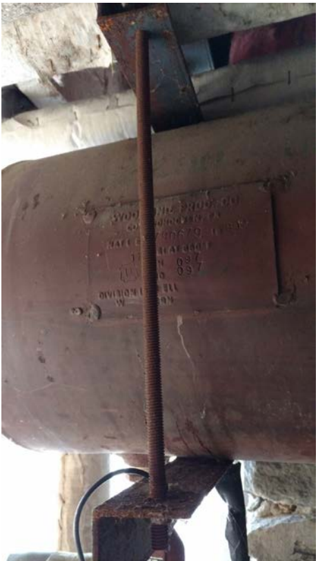
Figure 3.28 Chilled Water Expansion Tank Nameplate Data M5
