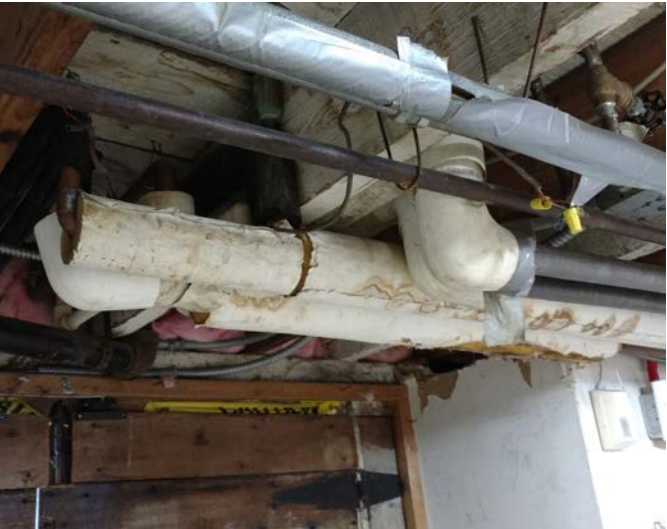
Figure 3.38 Rust on Heating Hot Water Piping & Damaged Insulation M37
