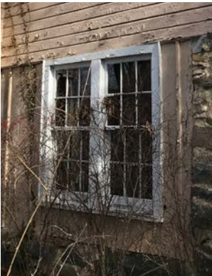
W0.7 Vegetation is Interfering with Window Function
