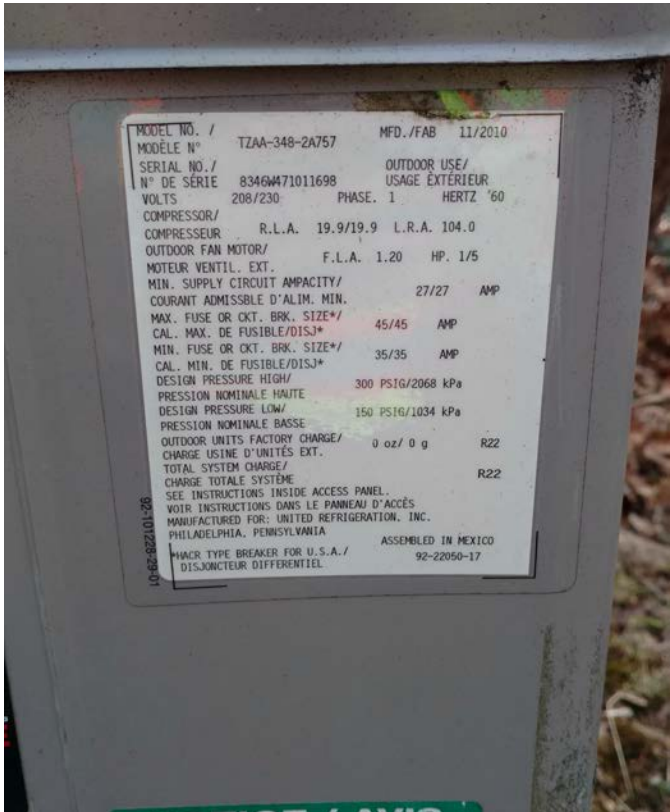
Figure 3.25 Chiller Air Cooled Condenser Nameplate Data M7
