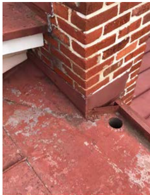
Peeling Paint at Upper Roof - Chimney C3 A14
