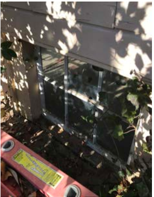
W0.1 Water Infiltration and Rot at Ground Plane
