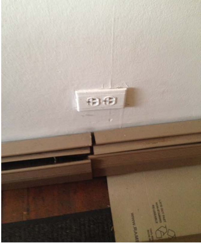
Figure 3.119 Receptacle located above baseboard heater E12
