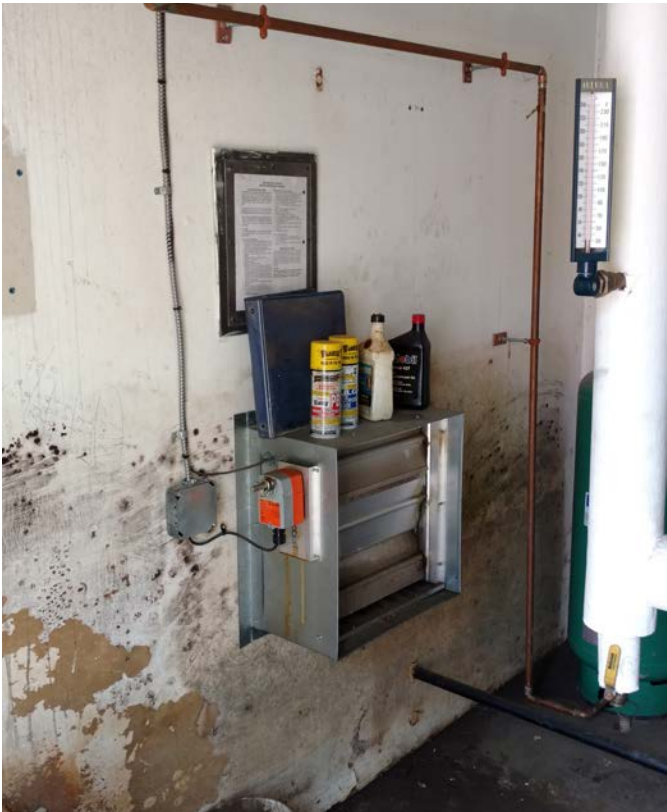
Figure 3.48 Boiler Shed Ventilation Damper and Actuator M15
