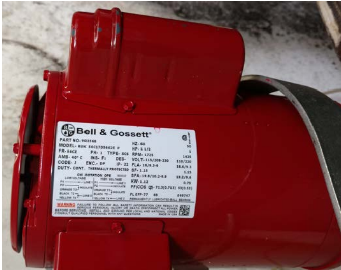
Figure 3.45 Heating Hot Water Inline Pump Nameplate Data M13
