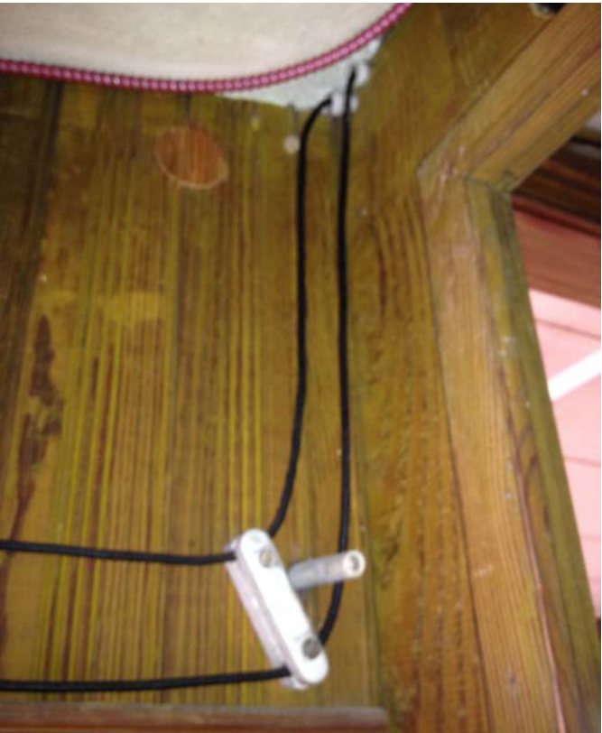
Figure 3.121 Obsolete knob-and-tube wiring E13
