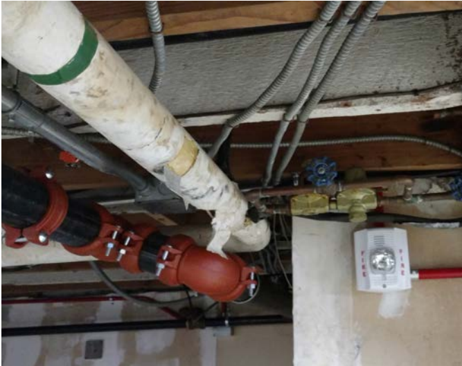
Figure 3.41 Chilled Water Piping with Torn & Water Damaged Insulation M39
