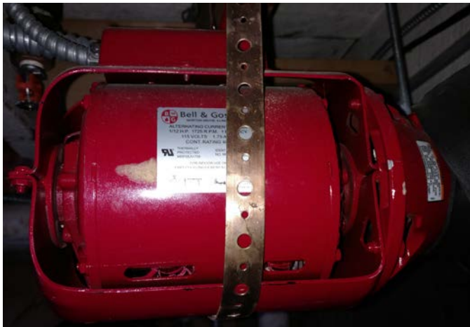
Figure 3.26 Chilled Water Inline Pump in Unfinished Basement M2
