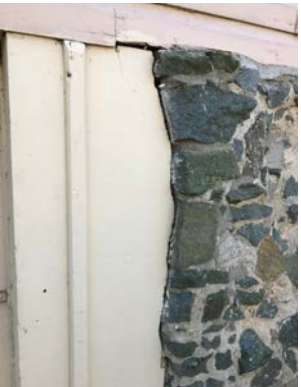
Masonry / Siding Joint Lacks Sealant
