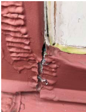
Cracked Flashing A9
