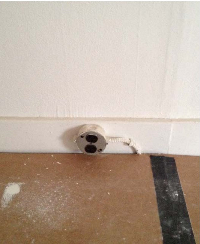
Figure 3.112 ADA compliance violation - device mounted too low
