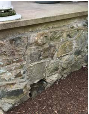
Damaged Masonry
