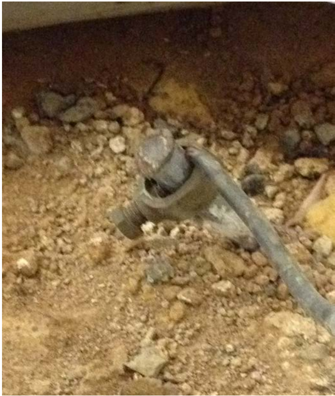
Figure 3.109 Insufficient grounding E6
