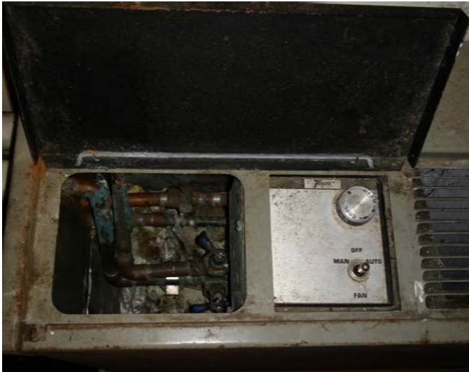
Figure 3.31 Fan Coil Unit Controls and Valving (Museum Collection Storage 006) M10
