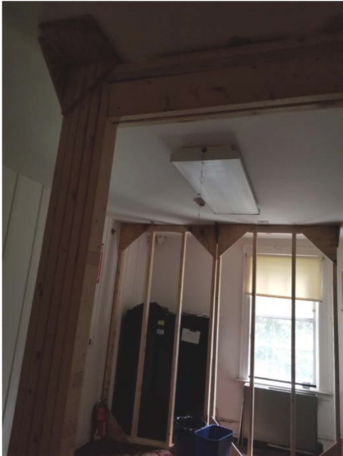
Figure 3.15 Structural Shoring in Office [106]
