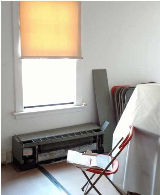
Figure 3.66 Four-pipe Fan Coil Unit serving Visitor Orientation 113 M19
