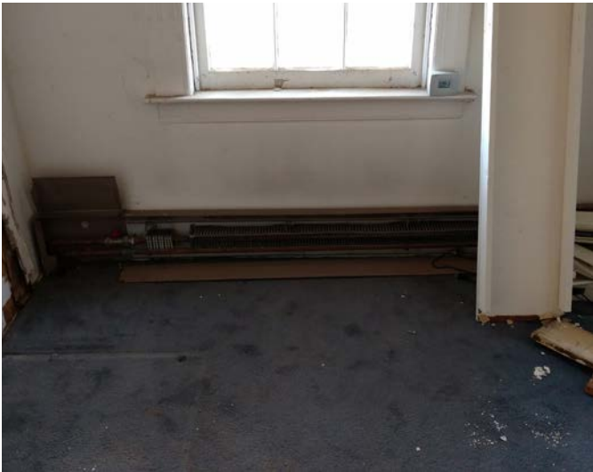
Figure 3.70 Hot Water Finned Tube Radiator serving Collection Storage 105 M21
