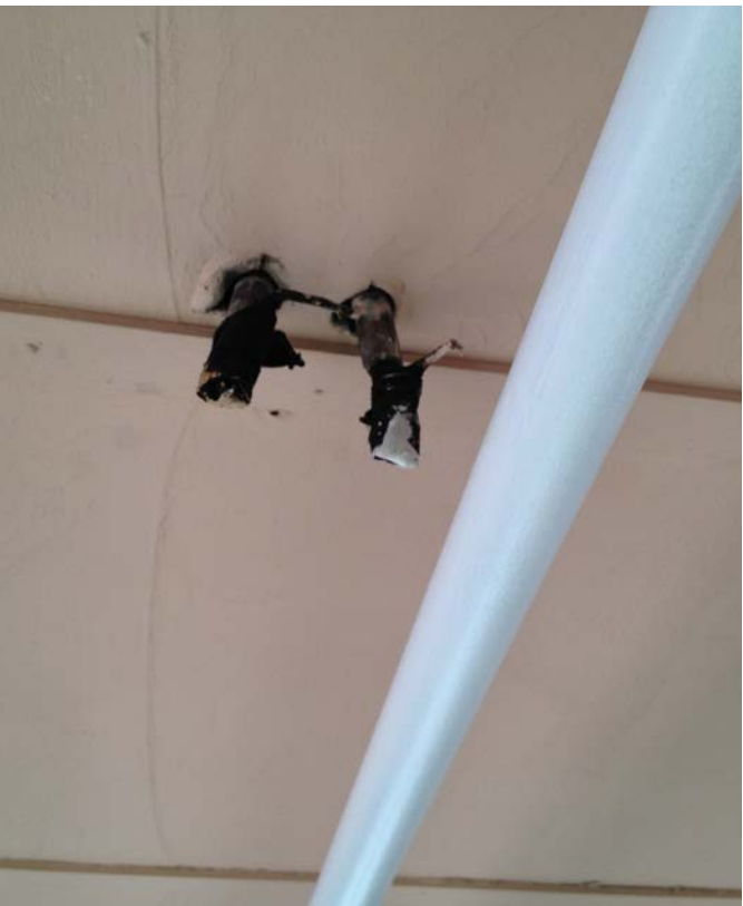
Figure 3.122 Obsolete knob-and-tube wiring E14
