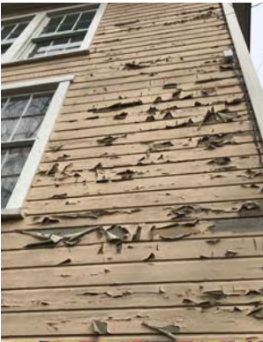
Siding has Peeling Paint
