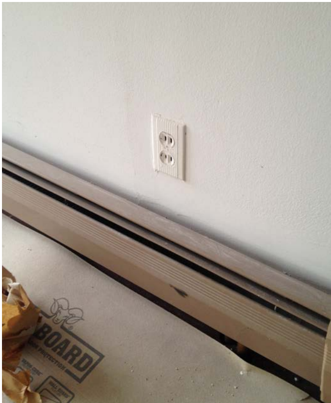
Figure 3.118 Receptacle located above baseboard heater E11
