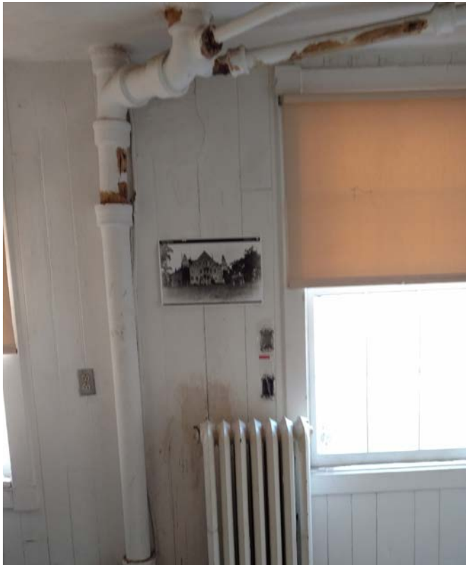
Figure 3.82 Damage on Sanitary Piping Insulation within Clara Barton’s Kitchen 111 P5
