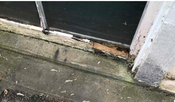
Water Damage to Sill and Window at Porch Roof A4
