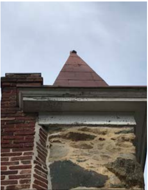
Tower Fascia has Peeling Paint
