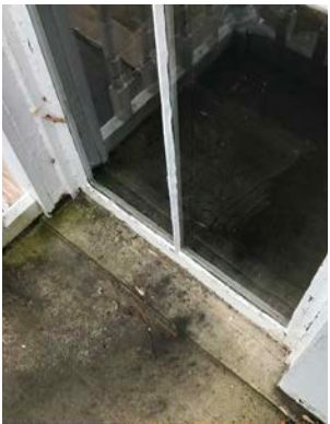
W3.13 Sill Damage Due to Low Slope of 2nd Floor Balcony
