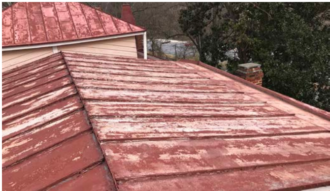
Peeling Paint at Upper Roof A18
