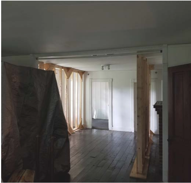
Figure 3.14 Structural Shoring in Rear Parlor [104]
