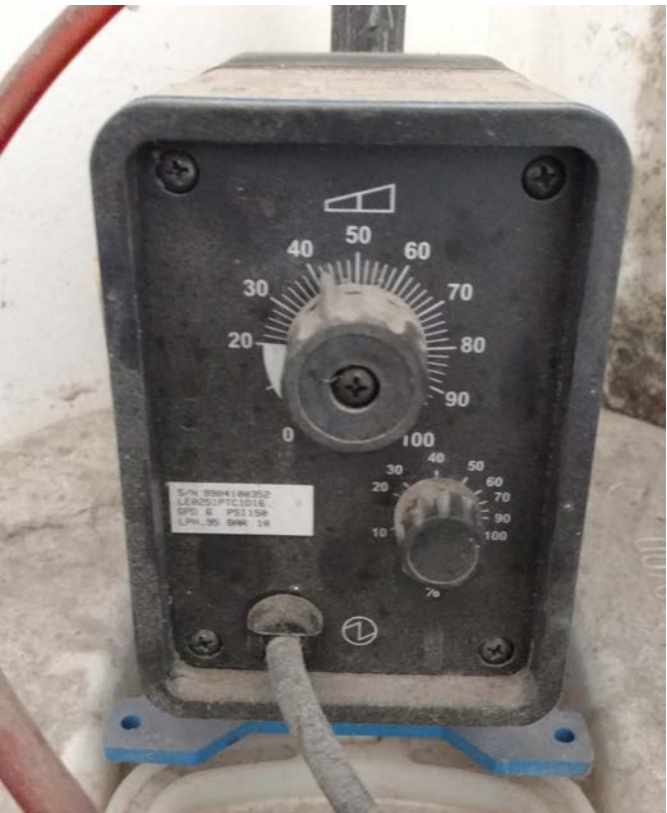
Figure 3.54 Electronic Metering Pump in Boiler Shed M16
