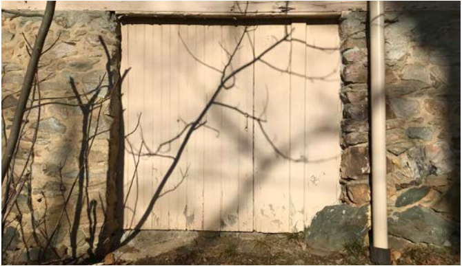
D0.2 Water Infiltration and Rot at Ground Plane. Peeling Paint.
