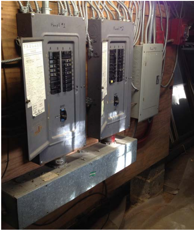
Figure 3.107 Service entrance conductors capacity is lower than the overcurrent devices at the service equipment; no surge protection devices E4
