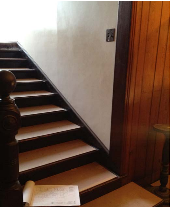
Figure 3.111 ADA compliance violation - device mounted too high E7
