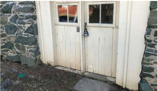
D0.4 Rotting at Ground Plane. Recently installed weather stripping interfering with function of the door. This door requires a comprehensive rebuild. This can be done using modern standards while retaining the historic look of the existing doors.
