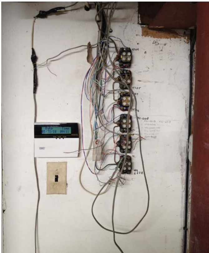
Figure 3.108 Telephone service entrance cable is exposed and unprotected; primary protection is obsolete and inadequate E5
