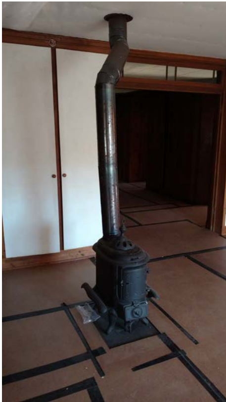
Figure 3.80 Stove with Built-in Custom Heater serving Center Red Cross Office 109 M27
