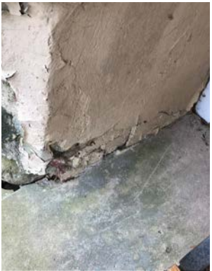
Damaged Exterior Stucco
