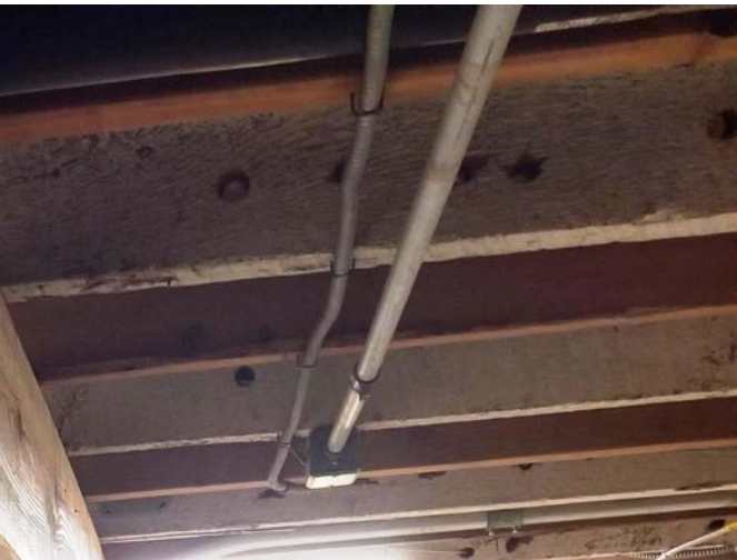
Figure 4.1 First Floor Joists (Painted White - Original; Unpainted - 1981 Strengthening)
