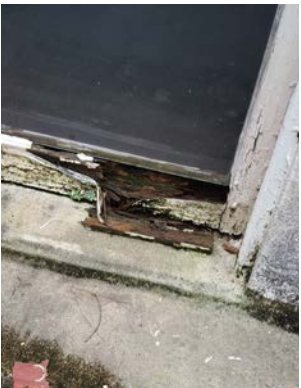
Damaged Window at 2nd Floor Balcony due to False Gable Roof Runoff
