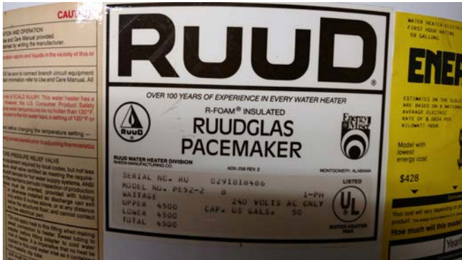
Figure 3.57 Electric Domestic Water Heater Nameplate Data P1
