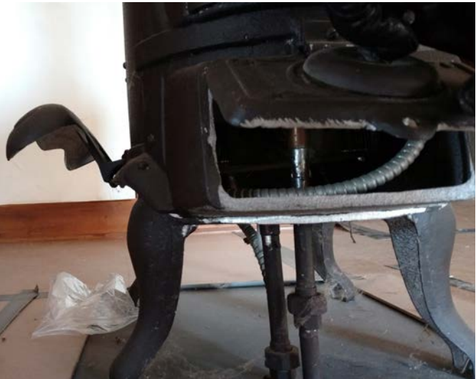
Figure 3.81 Room 109 Stove Built-in Custom Heater Hot Water Piping & Electrical Conduit M27
