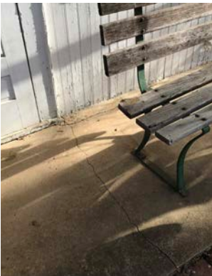
Concrete Patio is Cracked
