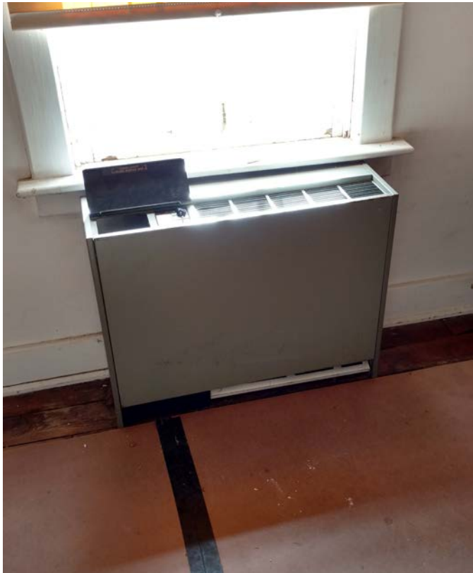
Figure 3.68 Four-pipe Fan Coil Unit serving Office 107 M20
