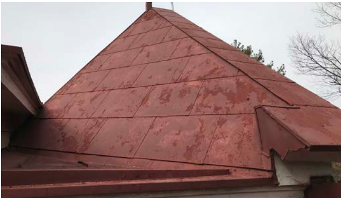
Peeling Paint at Rear of Front Gable A21
