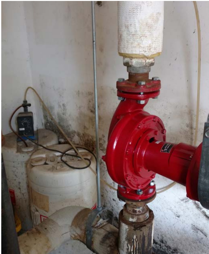
Figure 3.52 Heating Hot Water Inline Pump in Boiler Shed M13
