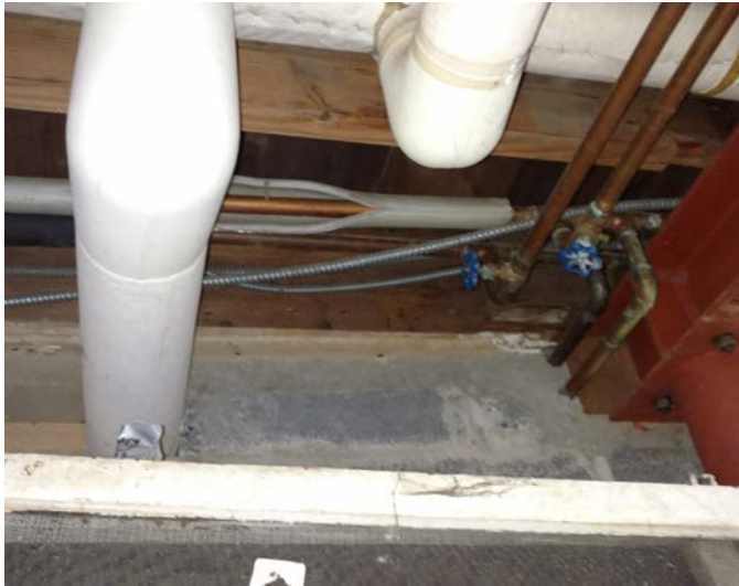
Figure 3.58 Uninsulated Domestic Water Piping & Valving Exhibiting Rust P2
