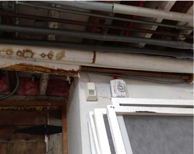
Figure 3.37 Rust on Heating Hot Water Piping & Damaged Insulation M37
