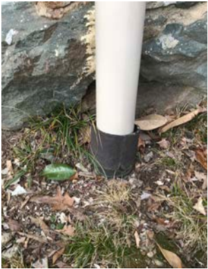
Drain Sleeve is Damaged
