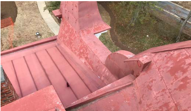
Peeling Paint at North Tower Roof A22
