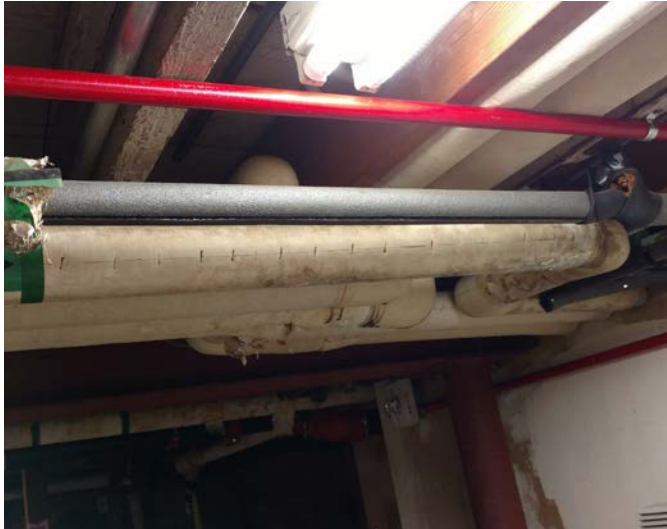
Figure 3.39 Chilled Water Piping with Mismatched Insulation Materials M38
