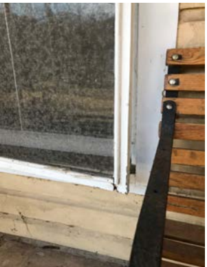
W1.25 Insect Screen Damaged
