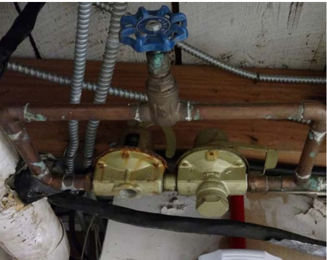
Figure 3.62 Chilled Water Make-up Backflow Preventer P4
