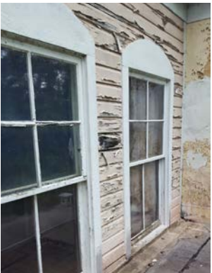
Damaged German Siding
