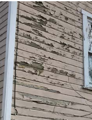
Siding has Peeling Paint
