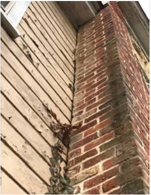
Chimney is Weathered and is Missing Sealant
