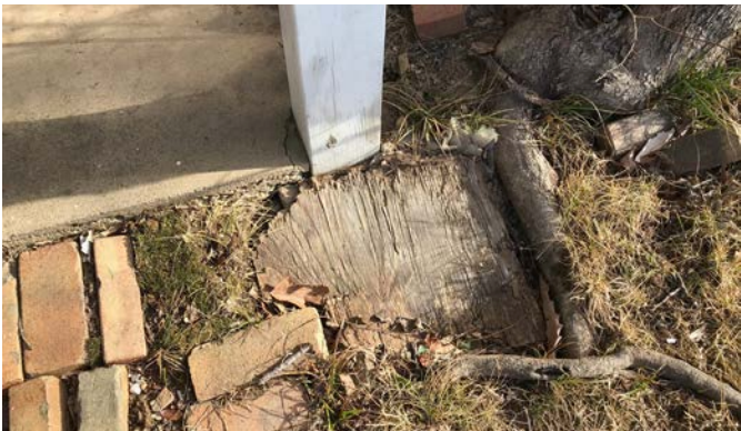
Hole in the Ground at the Column Base
