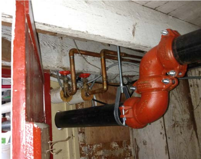
Figure 3.43 Missing Insulation on Heating Hot Water Piping M39
