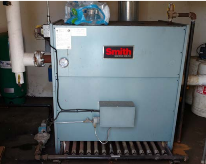
Figure 3.50 Gas-fired Hot Water Boiler in Boiler Shed M12
