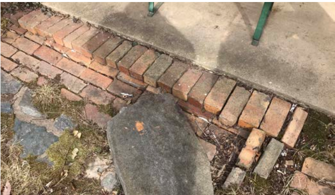
Brick Step has Missing Mortar and is Uneven
