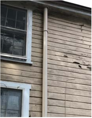
Siding has Peeling Paint
