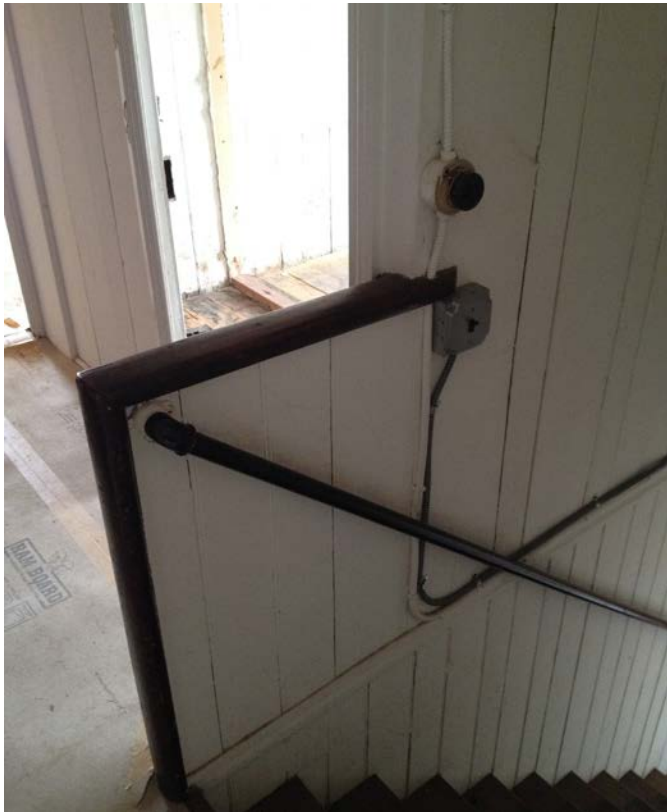
Figure 3.117 ADA compliance violation - device mounted too high or too low E10
