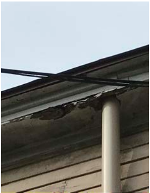
Eave Fascia is Damaged
