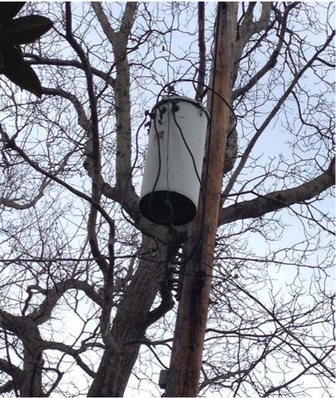
Figure 3.105 Electrical service capacity insufficient E2
