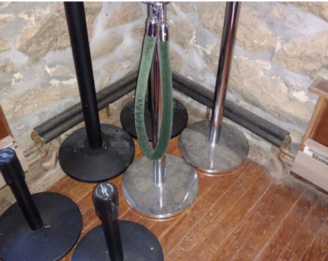
Figure 3.33 Hot Water Piping associated with Finned Tube Radiators in Museum Collection Storage 005 M11
