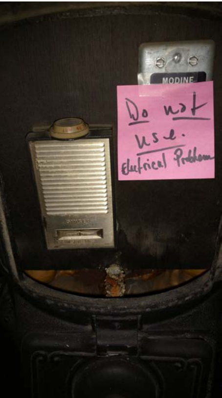
Figure 3.78 Vestibule 101 Stove Built-in Custom Heater Thermostat & Controls
