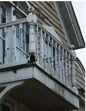
Damaged Balustrade at 3rd Floor Balcony
