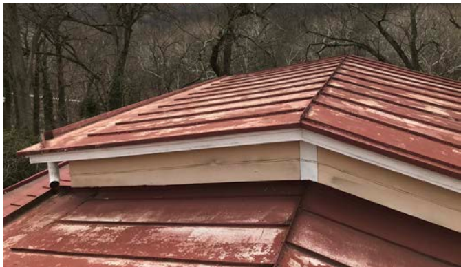
Peeling Paint at Upper Roof A17
