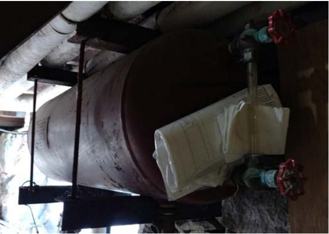
Figure 3.34 Chilled Water Expansion Tank in Unfinished Basement M5
