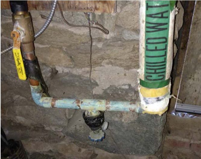
Figure 3.40 Chilled Water Piping with Calcium Build-up & Missing Insulation M38
