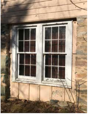
W0.6 Water Infiltration and Rot at Ground Plane
