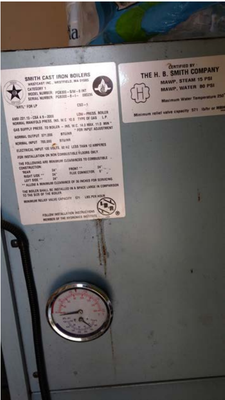
Figure 3.51 Gas-fired Hot Water Boiler Nameplate Data M12
