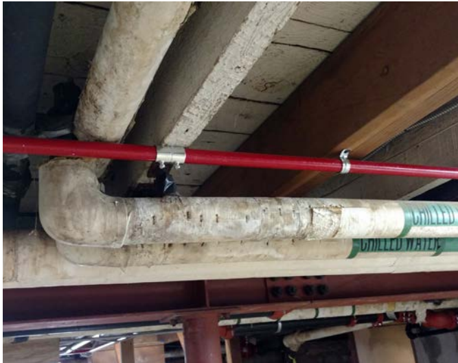
Figure 3.42 Chilled Water Piping with Water Damaged Insulation M39
