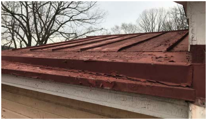
Peeling Paint at Upper Roof A15
