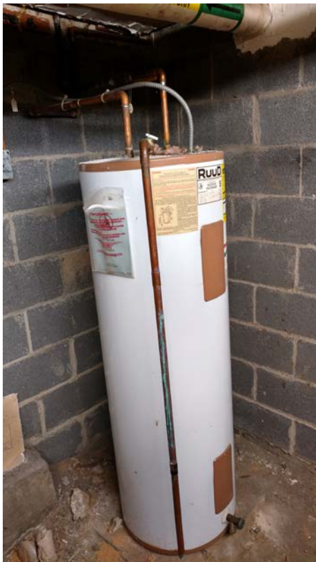
Figure 3.56 Electric Domestic Water Heater in Mechanical Room within Unfinished Basement
