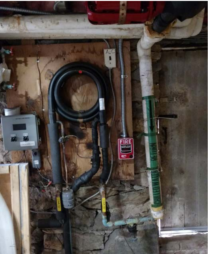
Figure 3.21 Chiller Evaporator Coil in Unfinished Basement M1
