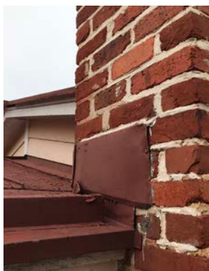
Cracked Flashing - Chimney C3 A11
