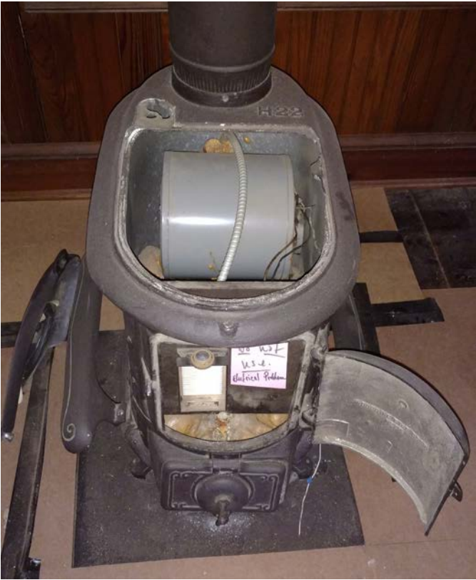
Figure 3.77 Stove with Built-in Custom Heater serving Vestibule 101
