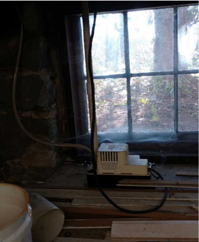
Figure 3.35 Condensate Pump and Associated Tubing M4
