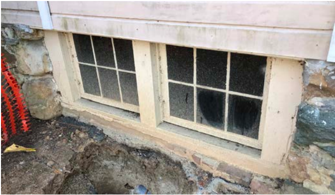
W0.17 Rotting at Ground Plane
