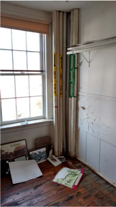
Figure 3.73 Heating Hot Water & Chilled Water Pipe Risers in Office 112
