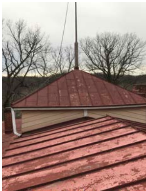
Peeling Paint at Upper Roof A10
