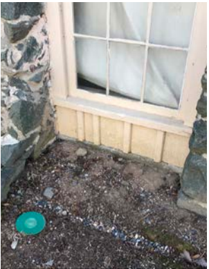
W0.12 Rotting at Ground Plane
