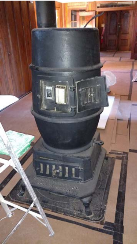
Figure 3.75 Stove with Built-in Custom Heater serving Hall 102
