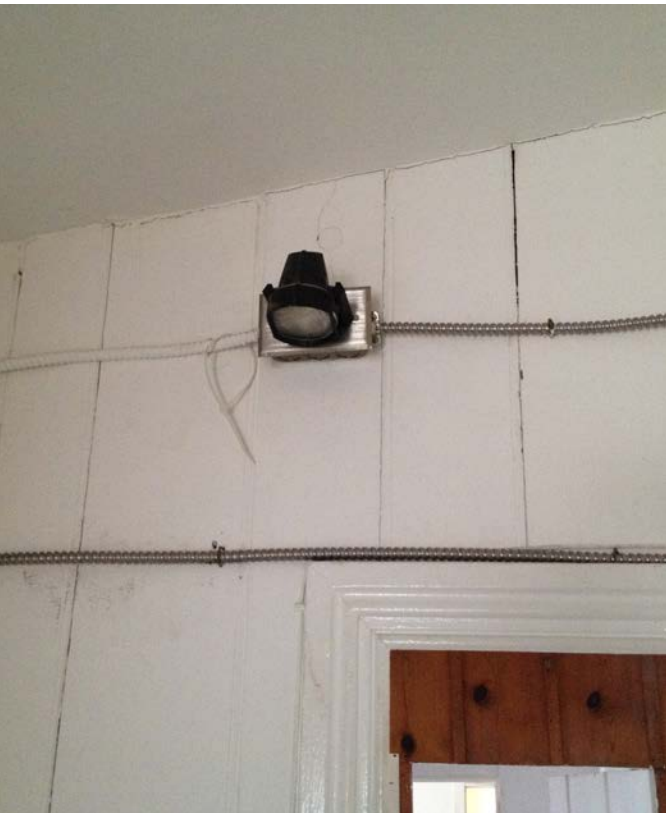
Figure 3.116 Emergency lighting and exit signage deficiencies E9
