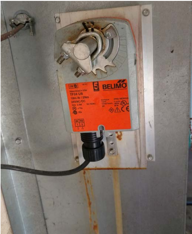
Figure 3.49 Boiler Shed Ventilation Damper Actuator M15
