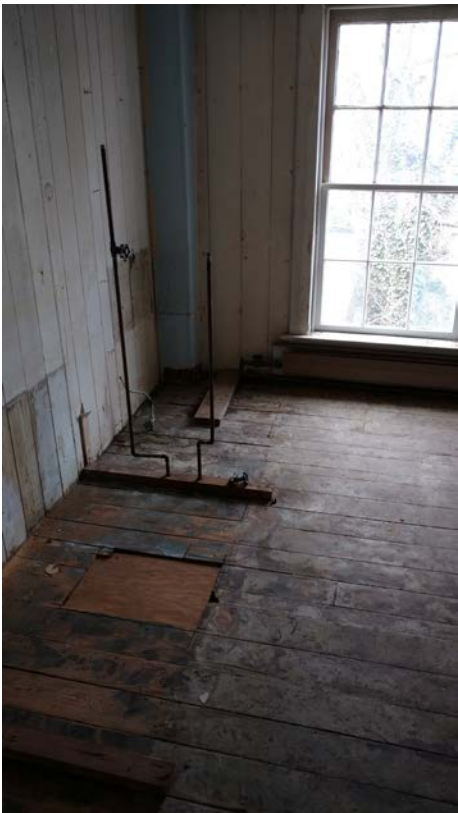
Figure 3.98 Domestic Water Lead Piping Exhibiting Rust within Clara Barton's Bathroom 210
