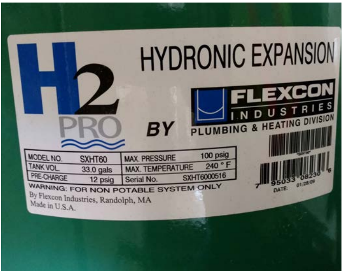
Figure 3.47 Heating Hot Water Expansion Tank Nameplate Data M14
