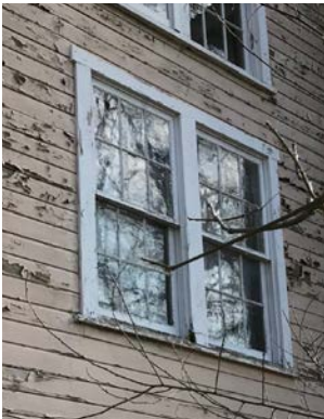
W1.14 Peeling Paint and Damaged Sill
