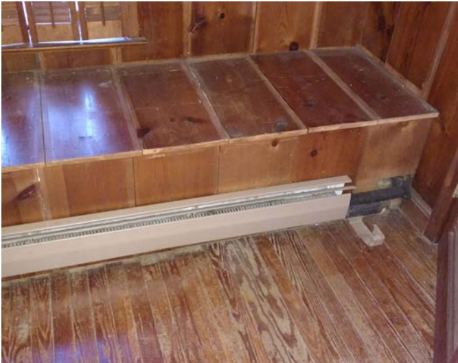
Figure 3.32 Finned Tube Radiator serving Museum Collection Storage 005 M11
