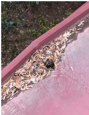
Obstructed Roof Downspout A8
