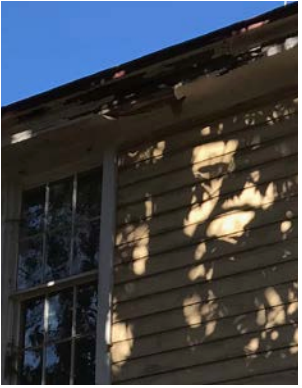
Eave Fascia is Damaged
