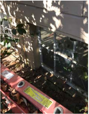
W0.2 Peeling Paint and Water Ingress
