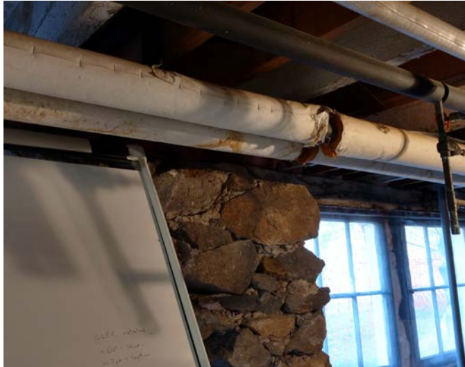
Figure 3.44 Damaged Insulation on Heating Hot Water Piping M39
