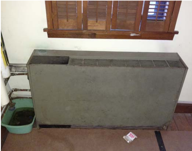
Figure 3.30 Four-Pipe Fan Coil Unit Serving Museum Collection Storage 006 M10
