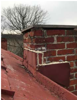
Flashing Cracked - Chimney C2 A12
