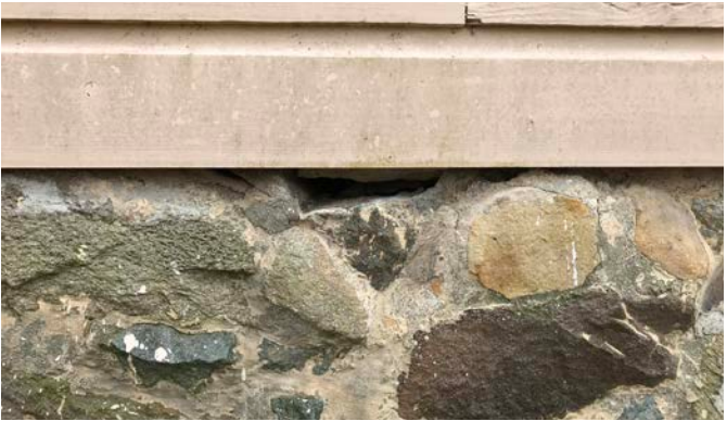
Damaged Masonry
