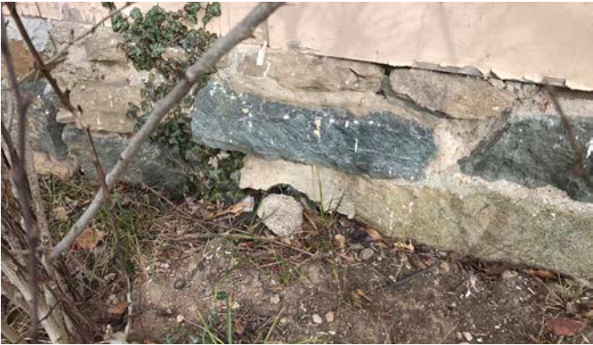
Damaged Masonry
