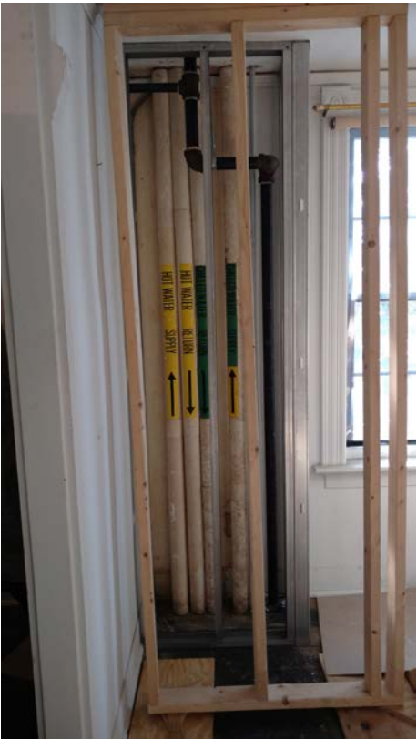
Figure 3.74 Heating Hot Water & Chilled Water Pipe Risers in Rear Parlor 104
