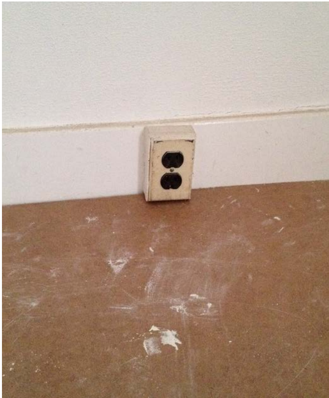
Figure 3.113 ADA compliance violation - device mounted too low
