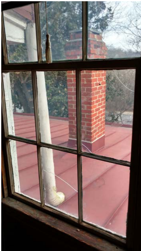
Figure 3.101 Metal Downspouts on Lower Roof (View from 3rd Level Windows)
