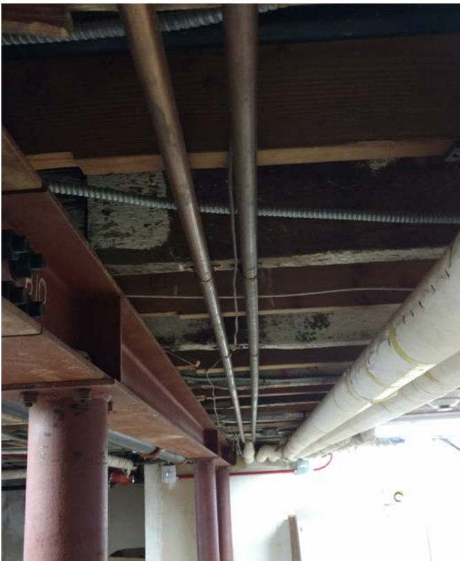
Figure 3.60 Uninsulated Domestic Water Piping P2
