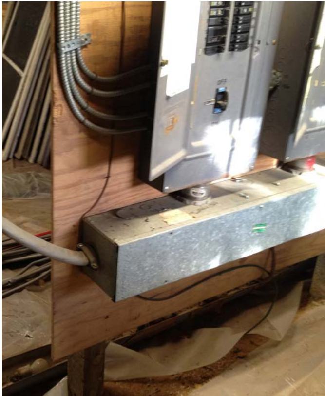
Figure 3.106 Service entrance cable is exposed and subject to physical damage E3
