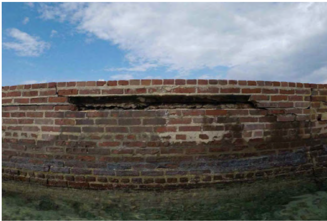
2 DEFECT TYPE 2 – ABOVE WATER LOSS OF BRICK/MORTAR NTS
