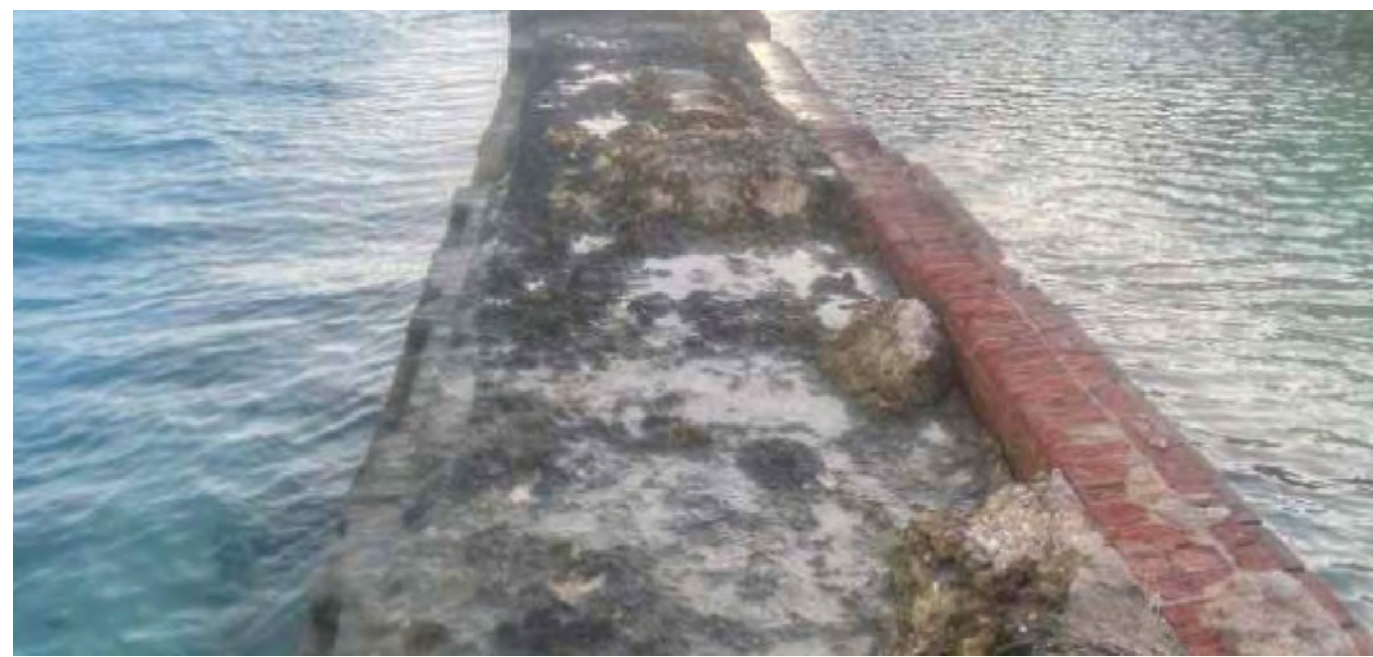
1 DEFECT TYPE 1 – LOSS OF WALKWAY CONCRETE NTS
