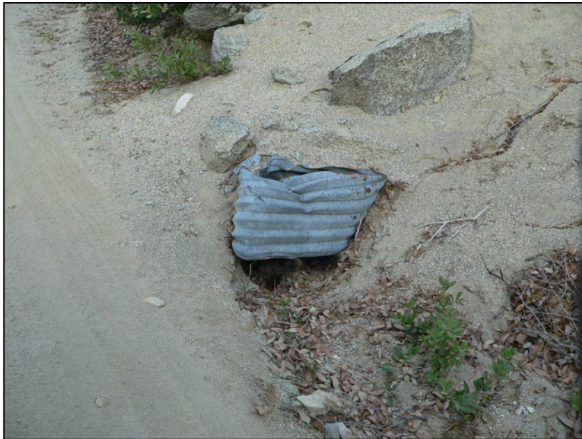
DEFERRED MAINTENANCE AT CRUSHED CULVERT ALONG SHASTA BALLY ROAD
