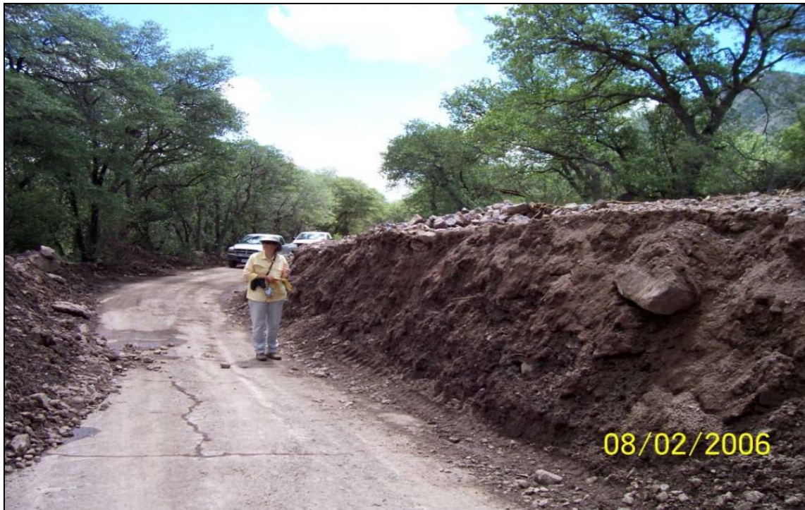
Figure 4 Picture illustrates the road damage caused to East Montezuma Canyon Road after the July 2008 flooding event. Photo taken looking east toward the visitor center and across two large historic culverts (not visible) that were plugged during the event.
