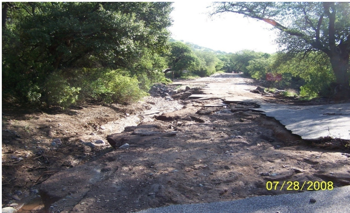
Figure 4 Picture illustrates the road damage caused to East Montezuma Canyon Road after the July 2008 flooding event. Photo taken looking east toward the visitor center and across two large historic culverts (not visible) that were plugged during the event.
