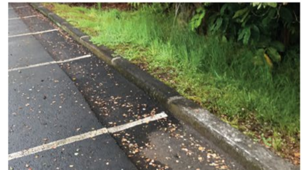
CURB - CONCRETE MATCH EXISTING CONCRETE CURB ON SITE IN TEXTURE, COLOR, AND USE OF SECTIONS WITH MORTAR JOINTS
