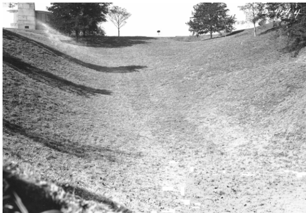
FIGURE 189. View looking northwest toward the Missouri State Memorial showing completed slope, November 7, 1935. These 1930s photographs illustrate the filling, grading, and sodding efforts conducted by the CCC. These images are an example of the many similar efforts conducted in numerous locations around the park at the time to correct erosional problems threatening roads and monuments. Agricultural activities had led to a lack of vegetative cover to protect against the loss of soil due to overland flow of stormwater. The CCC worked to protect the soil from further erosion through filling, grading, and sodding.
