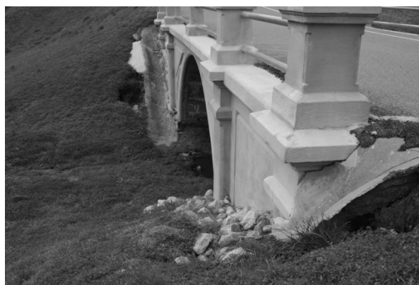
FIGURE 73. Erosion around the footings of historic Melan Arch Bridge No. 2 along Union Avenue north of Pemberton Avenue, looking southwest.
