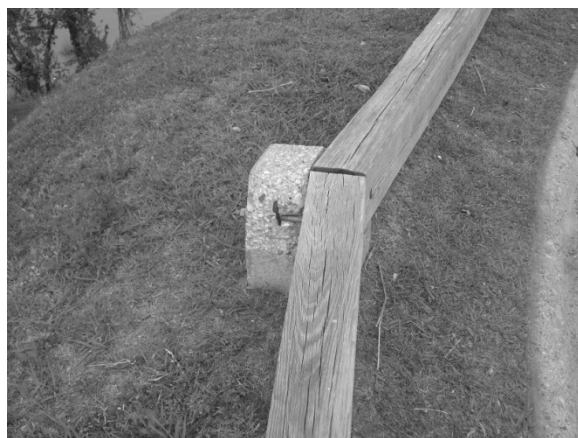
FIGURE 180. Portions of the timber guard rail along the Navy Circle access road have been damaged by cars.
