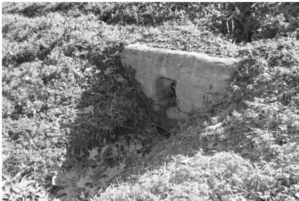
FIGURE 130. Other culverts within the park are made of brick, such as this outlet viewed looking east from the South Loop road near Fort Garrott.
