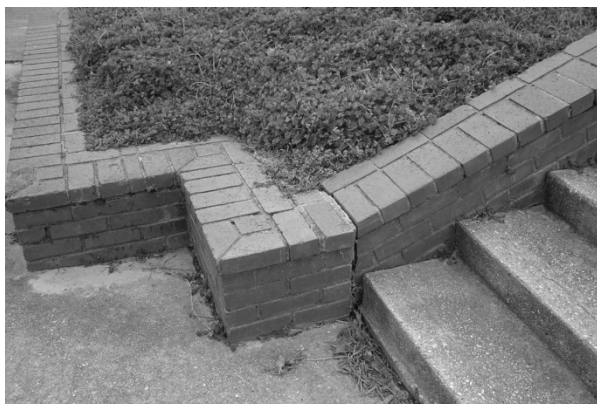
FIGURE 133. A brick retaining wall, edging the slopes of Fort Hill and forming the cheekwalls of the stairs which access the fortification.
