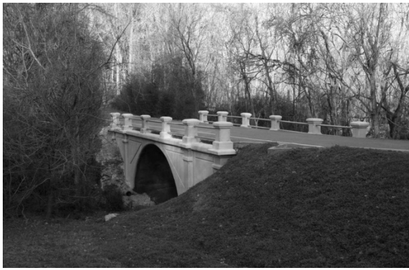
FIGURE 112. There are eight of the original nine Melan Arch bridges extant in the park. This historic, patented bridge-building style could span crossings without any intermediate supports. This bridge is just beyond the Memorial Arch on Union Avenue. This view is from the western side of Union Avenue, looking northeast.
