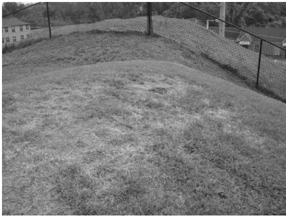
FIGURE 153. There are bald spots in the turf grass on the earthen fortification at Louisiana Circle that may lead to erosion.
