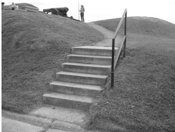
FIGURE 176. A flight of concrete steps leads up to the fort from the access road at Navy Circle. Erosion is undercutting the edge of the stairs.
