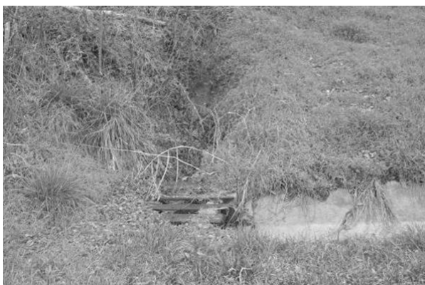
FIGURE 131. A CCC-era concrete gutter. Used on slopes for erosion control, these gutters were typically three feet wide and five to eight inches deep. This one is on the northwestern facing slope of Fort Hill.
