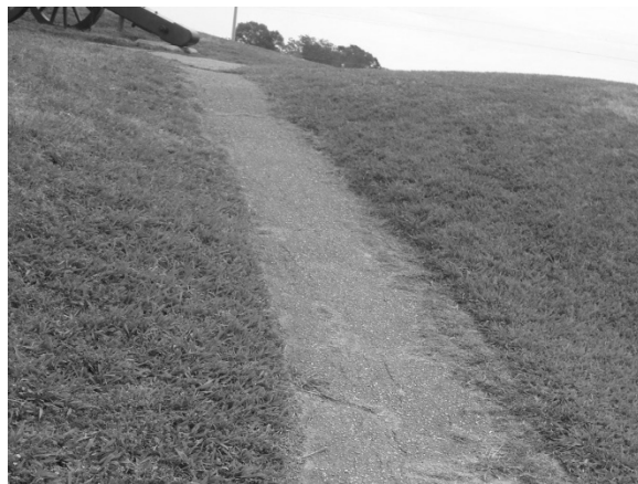
FIGURE 181. The asphalt on the walk leading to the top of the fortification at Navy Circle is cracking.
