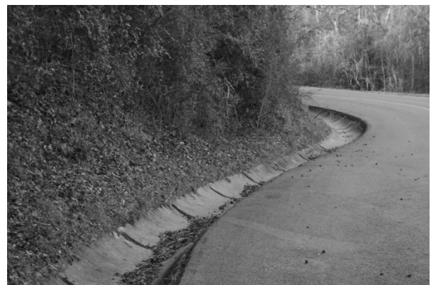
FIGURE 128. An elaborate system of curbs, gutters, and culverts control the overland flow of stormwater associated with roads and steep landforms within the park. Shown is a concrete swale along Union Avenue north of the Memorial Arch.
