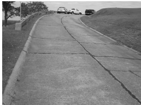
FIGURE 174. A concrete roadway encircles the knoll, providing visitor access to Navy Circle. Parking for approximately three cars is provided along the northern margin of the road. The road is edged by a low, rounded, mountable concrete curb and a concrete-post-and-wood-timber guard rail.
