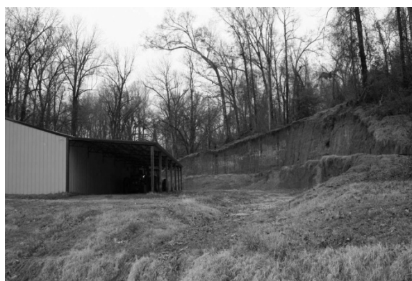
FIGURE 74. A borrow pit behind the maintenance complex, north of the visitor center, from which fill is used to repair erosion, an ongoing maintenance concern at the park.
