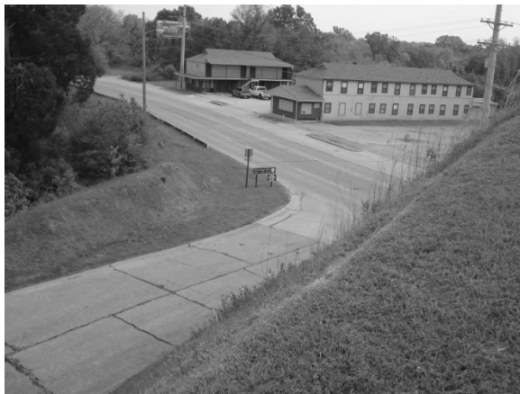
FIGURE 151. The concrete paving at Louisiana Circle that is cracked has been patched with a black asphaltic material that contrasts with the color of the paving.
