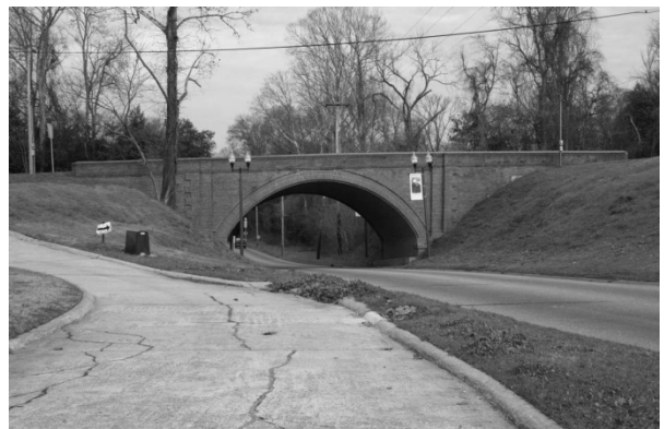
FIGURE 114. The Halls Ferry Road Bridge, from South Confederate Avenue, looking southwest. Composed of a single reinforced concrete arch span with brick facing, it is the only bridge of its kind in Mississippi. It is now on city-owned property.
