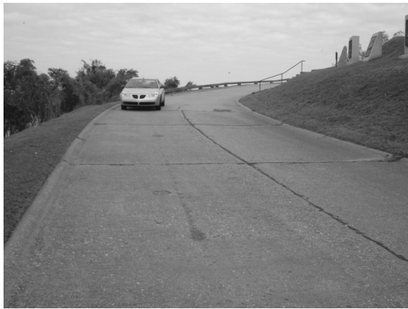
FIGURE 144. A concrete road circles around the base of the fortification at Louisiana Circle edged by rounded, mountable curbing and a guardrail composed of concrete posts and timber rails along its western margin.
