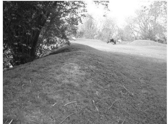
FIGURE 168. There are bald spots in the turf grass on the earthen fortification at South Fort that may lead to erosion.
