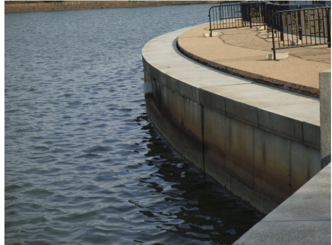
Photograph 4: The historic facing stones and capstones along the seawall are key features at the site. The facing stones and capstones would be removed prior to construction and replaced when the project was complete.
