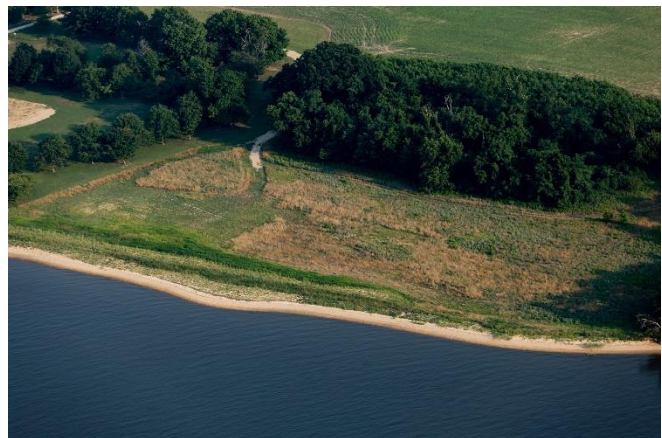
Figure N-2-1. Erosion is a natural process, but sometimes it is necessary to protect property from excessive erosion, like occurred (top) with Hurricane Isabel in 2003. Often the shoreline in or near developed areas is hardened – or “armored” – against erosion using bulkheads, revetments or riprap (middle). The use of softer approaches – such as the living shoreline (bottom) seen from the air – are becoming more common. Living shorelines protect against excessive erosion while providing ecological functions like habitat. Photos: Chesapeake Bay Program
