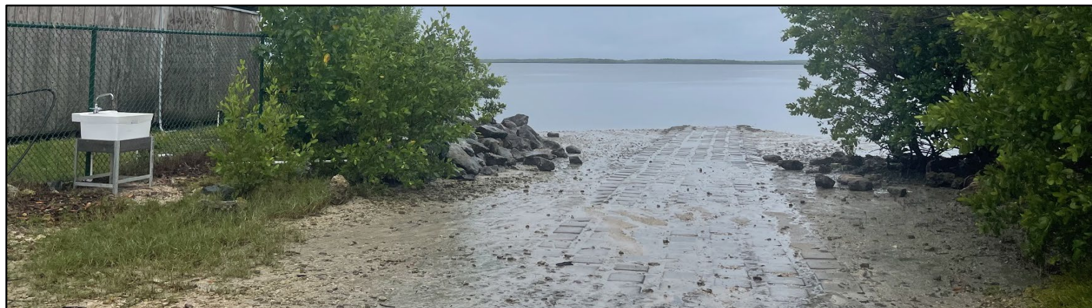
The deposition of sediment have filled in the marina basin, access channels, and canoe/kayak launch/NPS administrative boat ramp making them unusable during low tides and/or inefficient.
